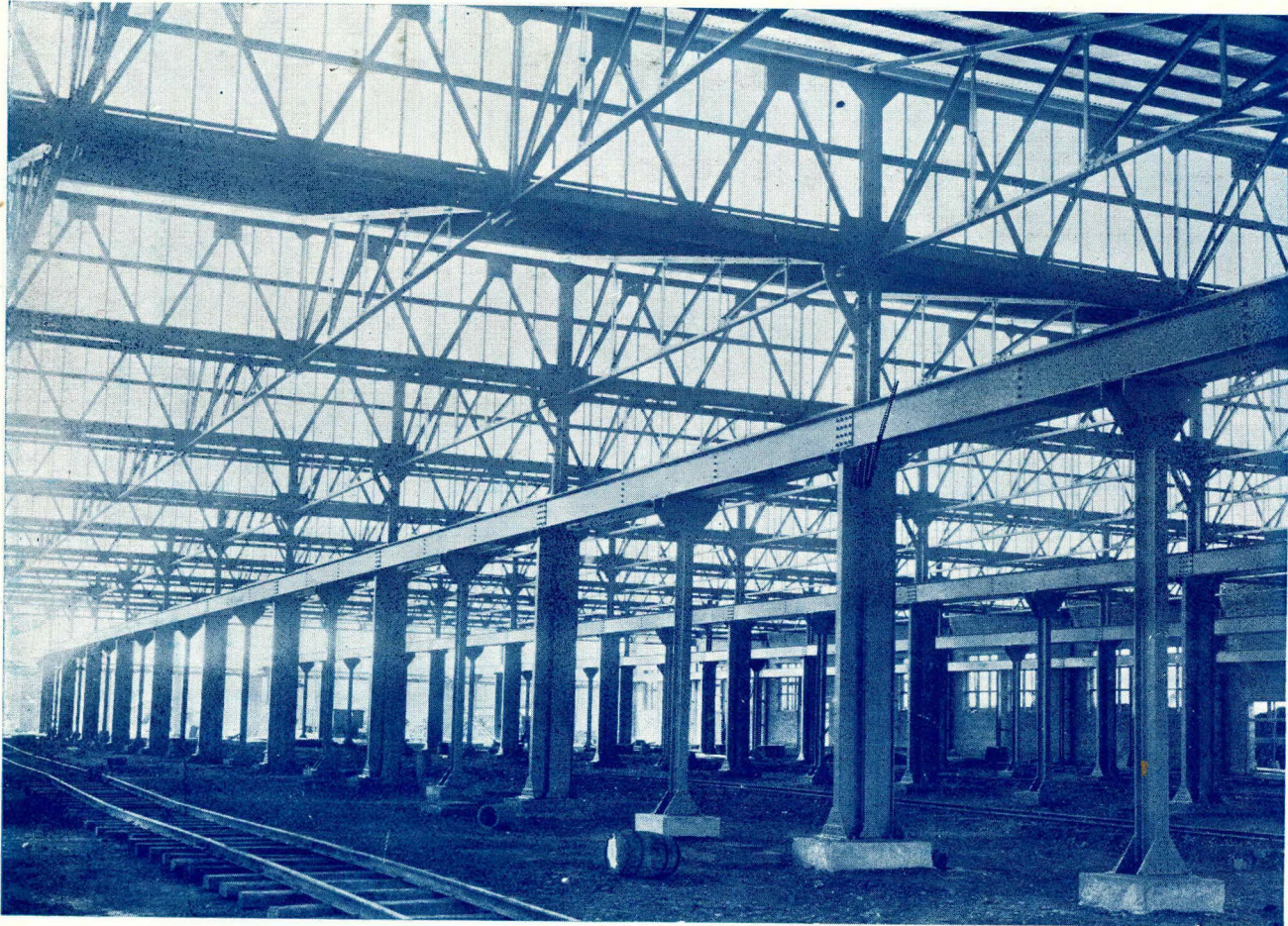
Internal View New Wagon Shops, S.A.R., Maritzburg. Total weight of structural steelwork nearly 1,000 tons. Supplied and erected by us complete.
