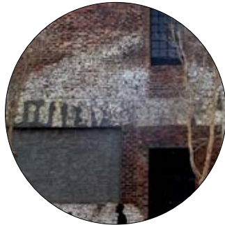
Brick variations and infills on Van Beek Street.
