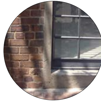
Grey plastered surrounds of window on Fox Street.
