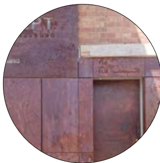
Corten clad wall and door at The Urban Fox on Fox Street.
