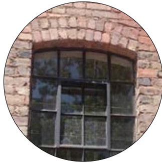
Arched brick-on-edge window sill on Fox Street.
