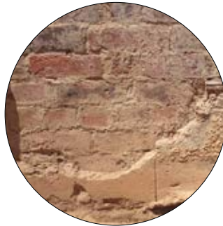
Plaster scraped off to reveal brickwork underneath on Fox Street.
