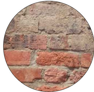
Brick variations and plaster on Fox Street.
