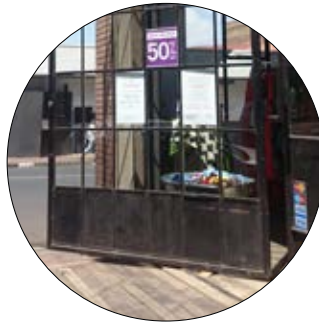
Large pivot opening steel doors to clothing store on Main Street.
