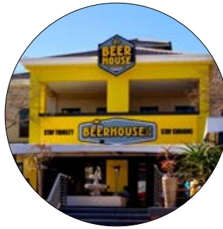
The prominent entrance to the Beer House in Fourways.
