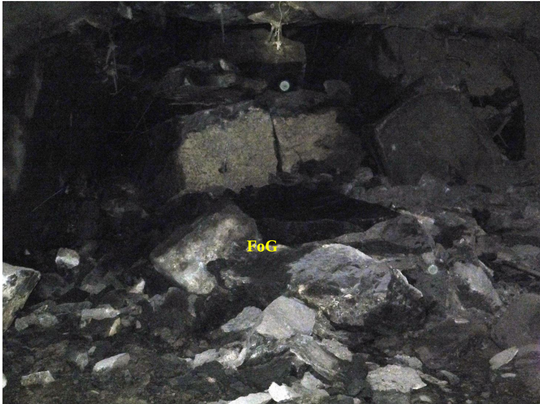
Figure 14: Fall of ground at the top of switchback 1
