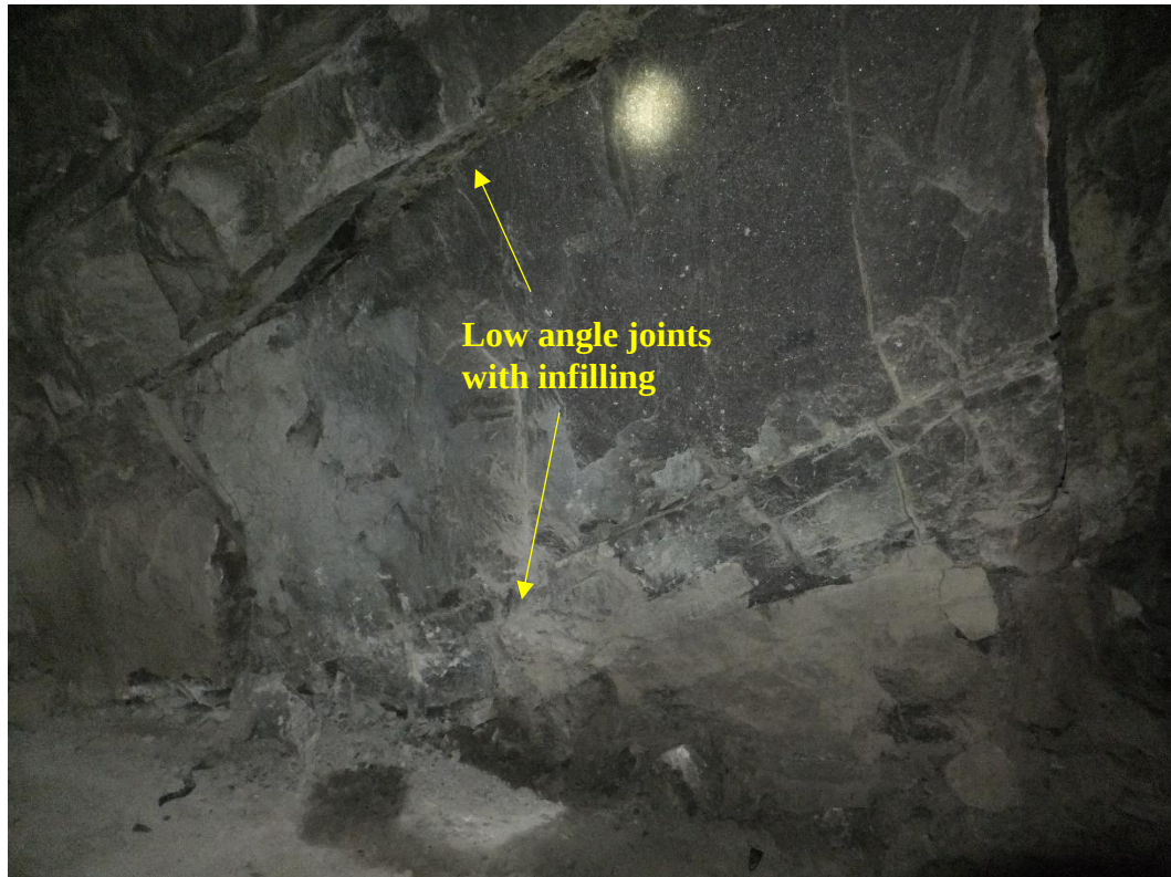
Figure 13: Existing low angle joints with infilling
