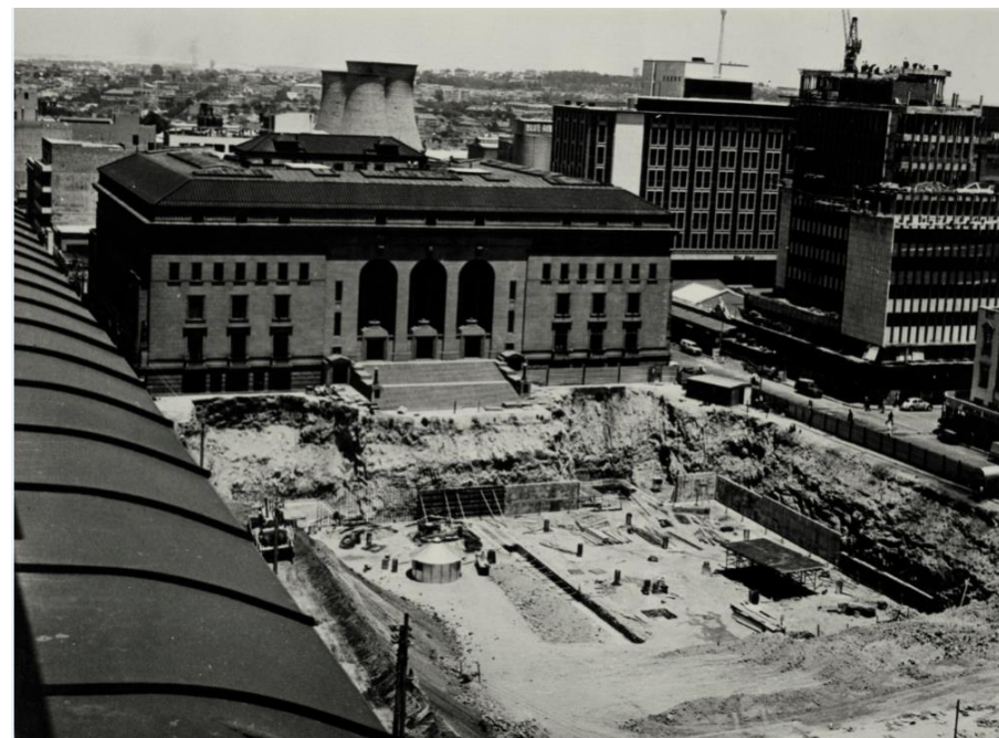
Image 49: Constructing the basement to be positioned underneath the Square, 1965 (Museum Africa Archives, 1965)
