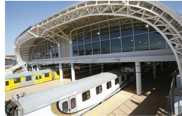
Image 21: Metrorail Trains at Park Station (Muchave, 2014)
