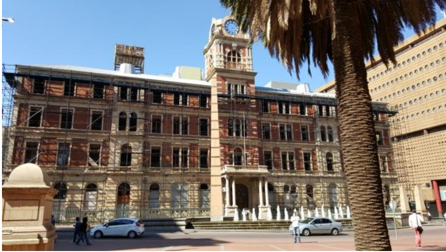
Image 65: Restoration efforts on the Rissik Street Post Office (Author, 2016)
