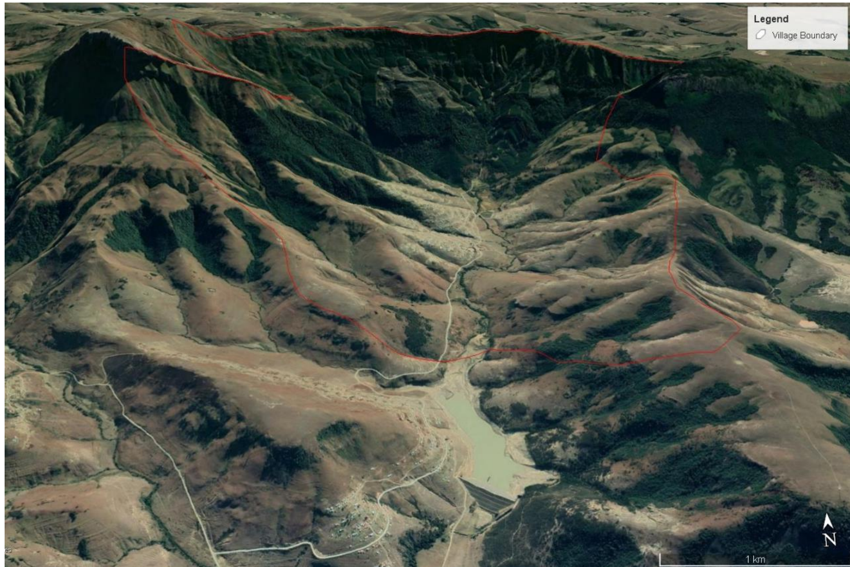
Figure B.7: Enlarged satellite image of Cata depicting slope (elevation exaggeration of 2) (Google Earth)
