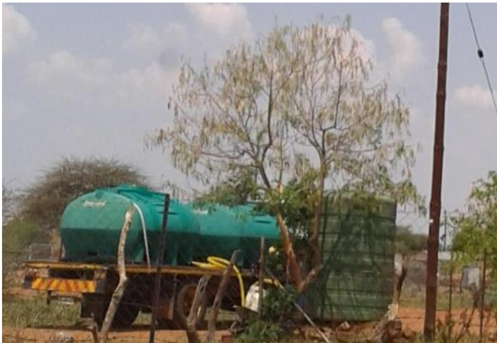
Figure 18: A water truck at a water point in Makapanstad pouring the water into stationary tank
