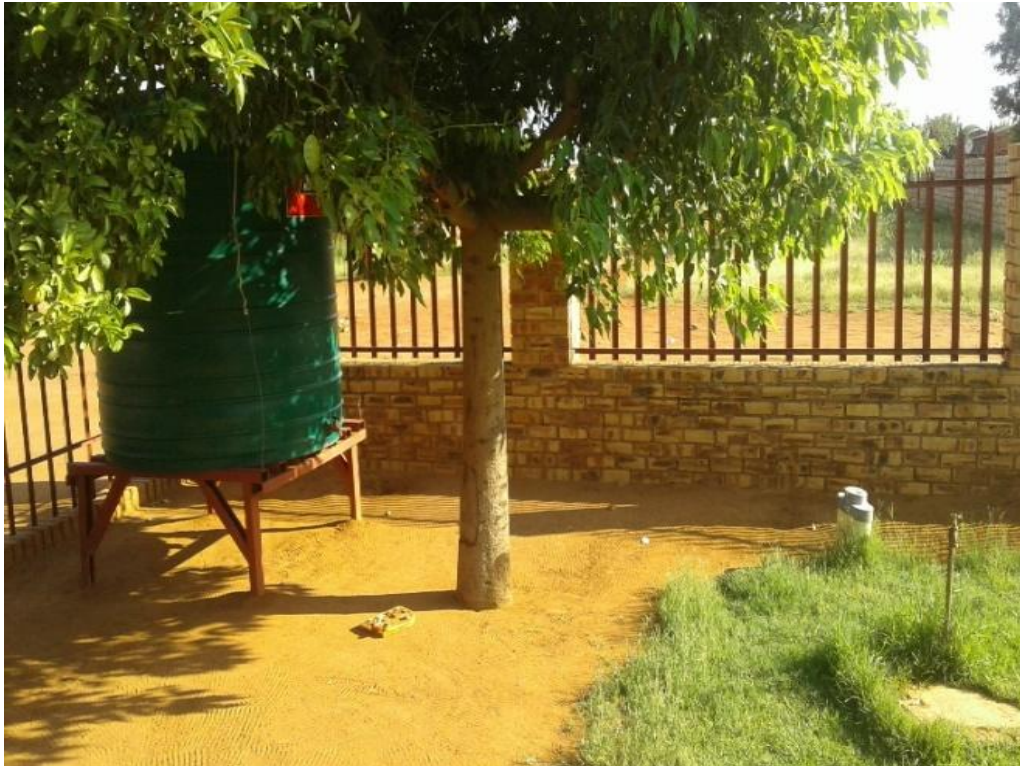
Figure 24: A yard in Carousel View displaying a tank to store water, a water tap and meter
