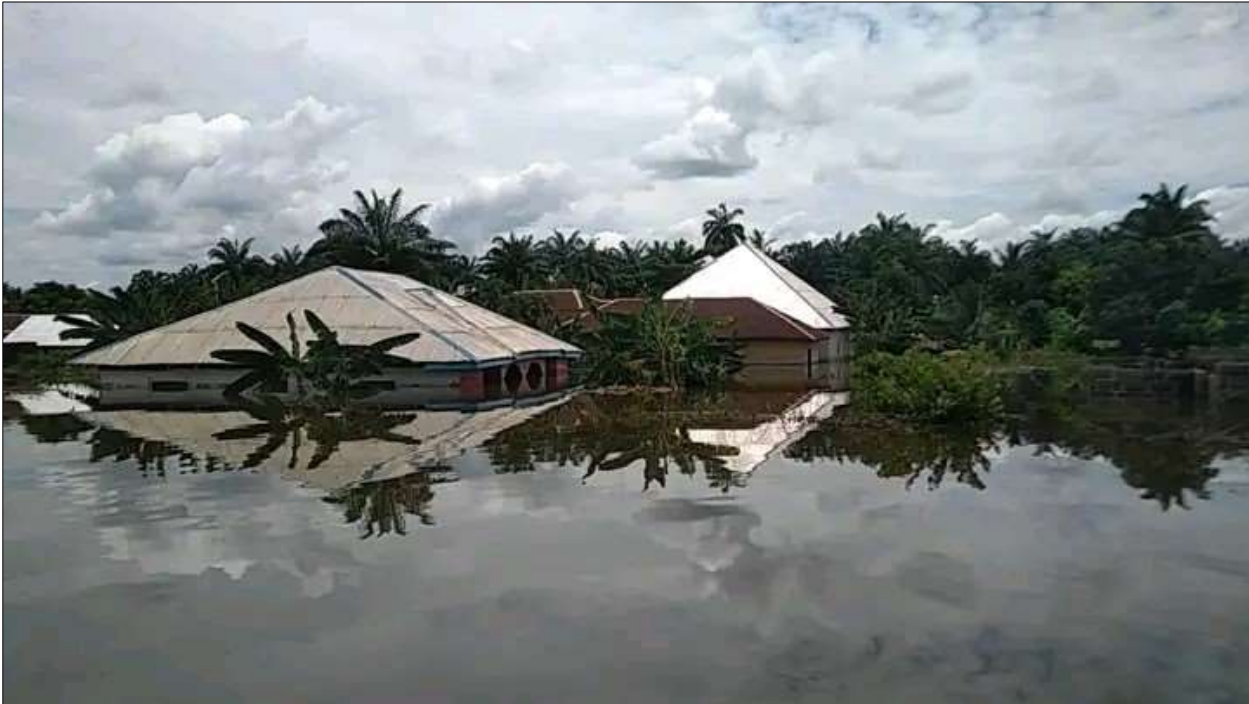
Figure 5.9: Flooded homes in Egbema caused by the October 2022 flood event
