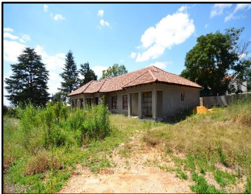
Image 10; Abandoned newly constructed home, Vredefort
