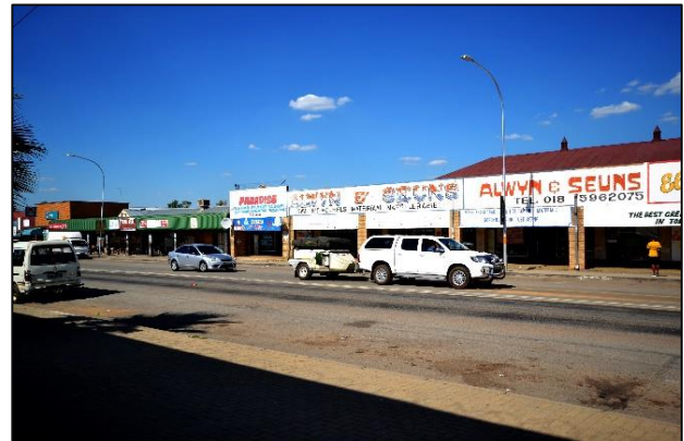
Figure 37: Street Scape in Wolmaransstad, North West
