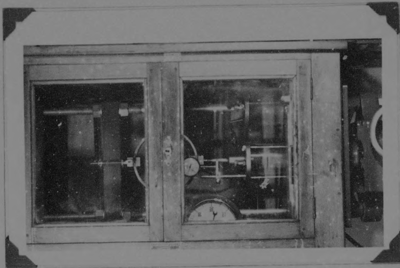
FIG 20 - OUTSIDE VIEW OF TEMPERATURE CONTROL CHAMBER ENCLOSING THE TEST BED
