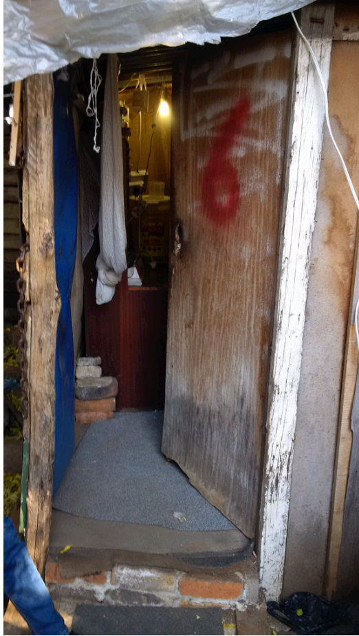
Figure 3.7: Doorway to a backyard room. (Source: MVP, 2020).
