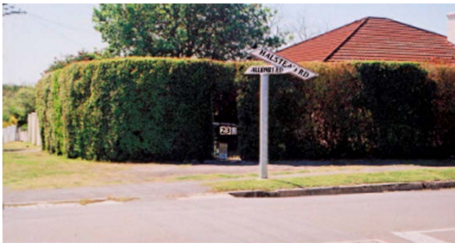
Photograph 1: The Lynette Elliot Frail Care Home
