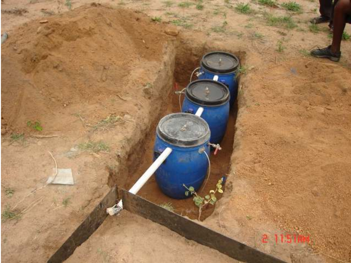
Figure 3.3: Series of runoff collection containers
