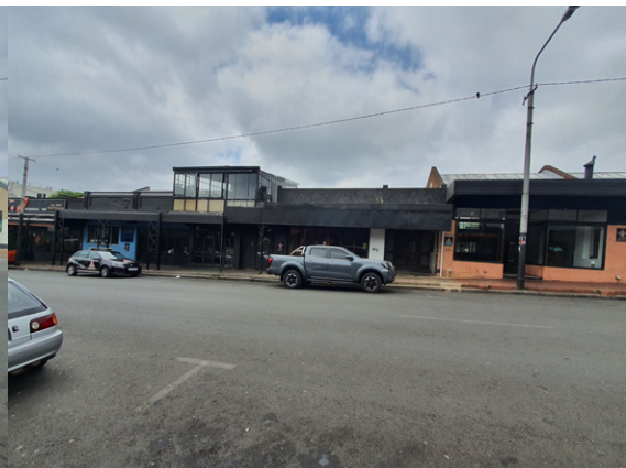
Site Photo - West - 7th Street figure 9.28: Site Photo, by Author (2023)
