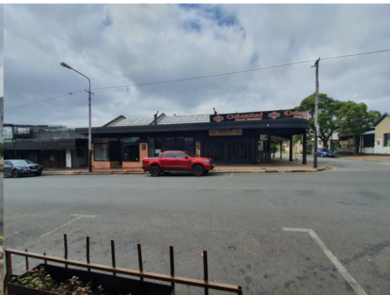
Site Photo - West - 7th Street figure 9.27: Site Photo, by Author (2023)
