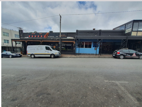
Site Photo - West - 7th Street figure 9.29: Site Photo, by Author (2023)
