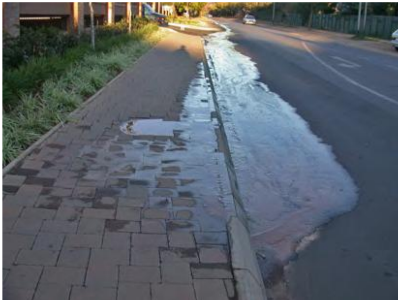
Figure 4: Physical Leakage, (Mckenzie et al., 2012)
