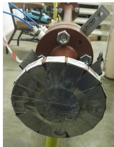
1. Meter run exit sealed
