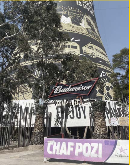
Figure 32 Orlando Towers Entrance. (Author, 2021)
