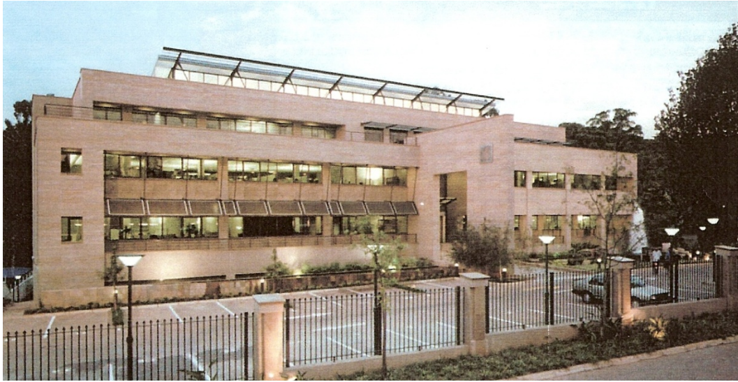
Figure B.3.01 MRe Offices – view of main entrance to building (Stauch Vorster MOM, 1998:1)
