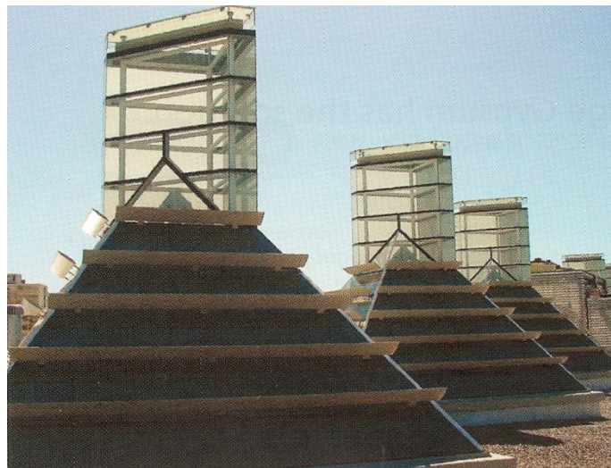
Figure B.4.12 BP Offices – close-up view of roof lanterns on roof (Noir and Roos, 2005:36)
