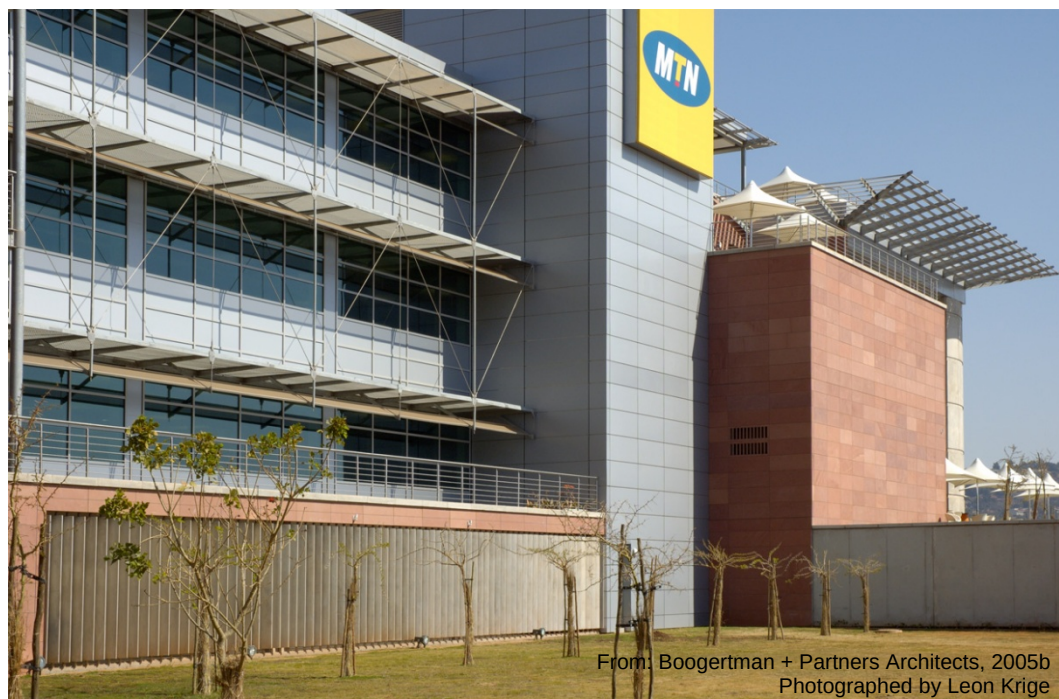
Figure B.2.11 MTN Offices – view of north façade with shading devices (Boogertman + Partners Architects, 2005b)
