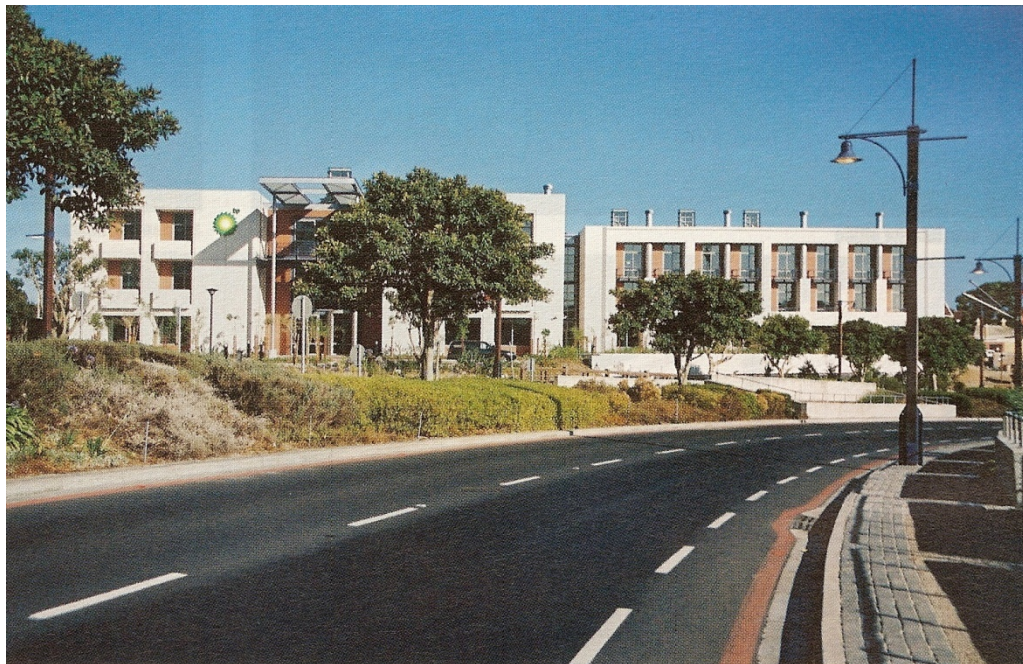
Figure B.4.02 BP Offices – view of building seen approaching from Dock Road (Kruger Roos Architects, 2004:90)
