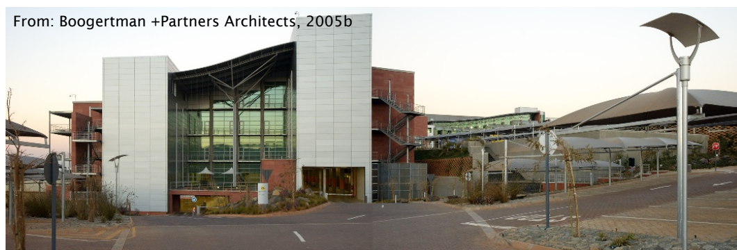
Figure 4.04 West elevation of the MTN Building
