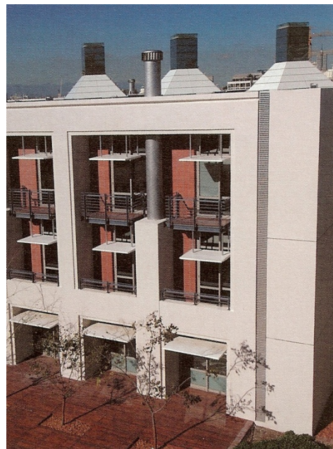
Figure B.4.05 BP Offices – view of green building design features (Digest of South African Architecture, 2006:137)
