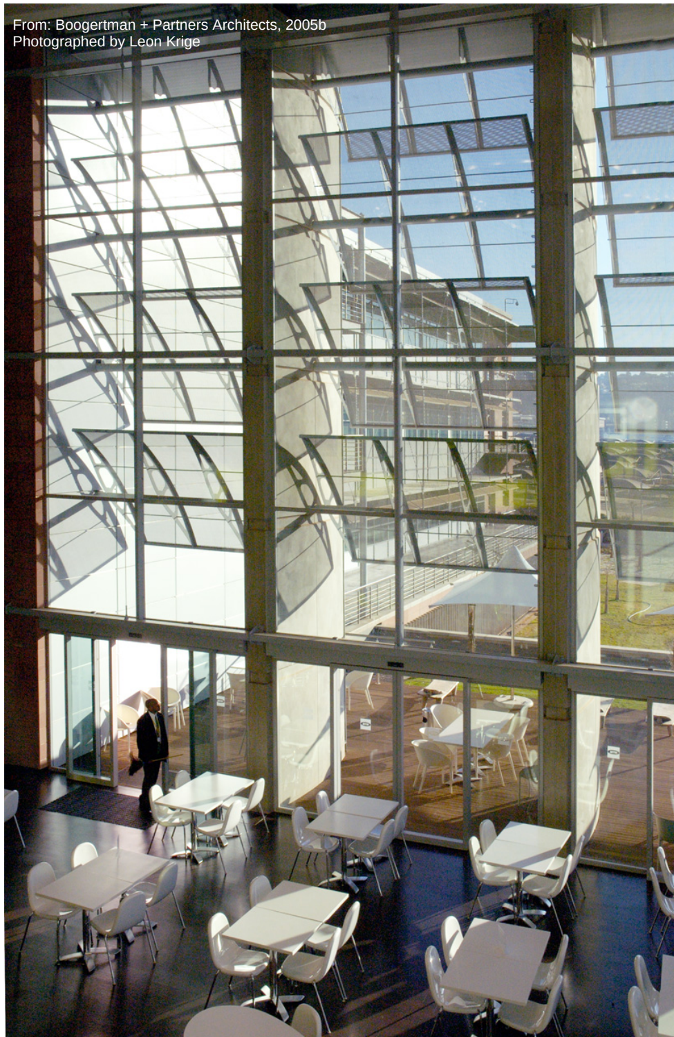
Figure B.2.16 MTN Offices – view of food court interiors showing shading devices on west facade (Boogertman + Partners Architects, 2005b)
