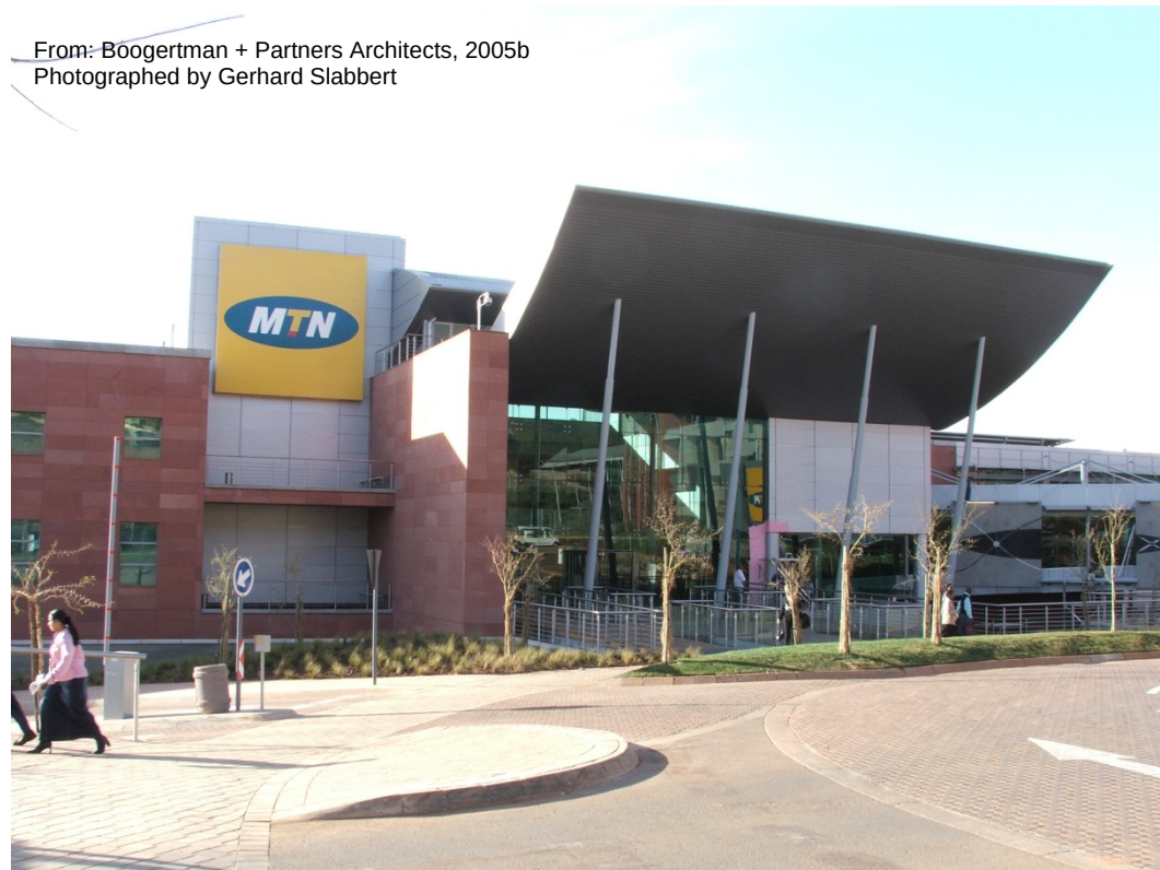
Figure B.2.10 MTN Offices – view of main entrance (Boogertman + Partners Architects, 2005b)
