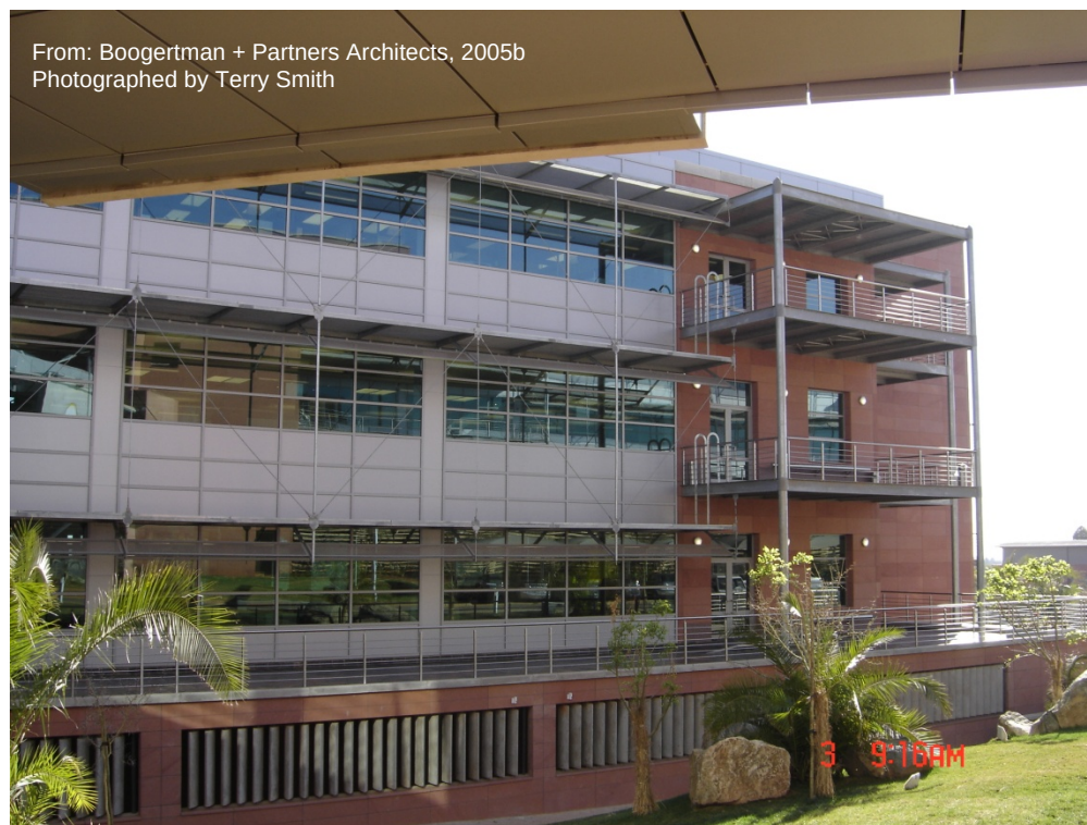
Figure B.2.13 MTN Offices – view of south façade (Boogertman + Partners Architects, 2005b)
