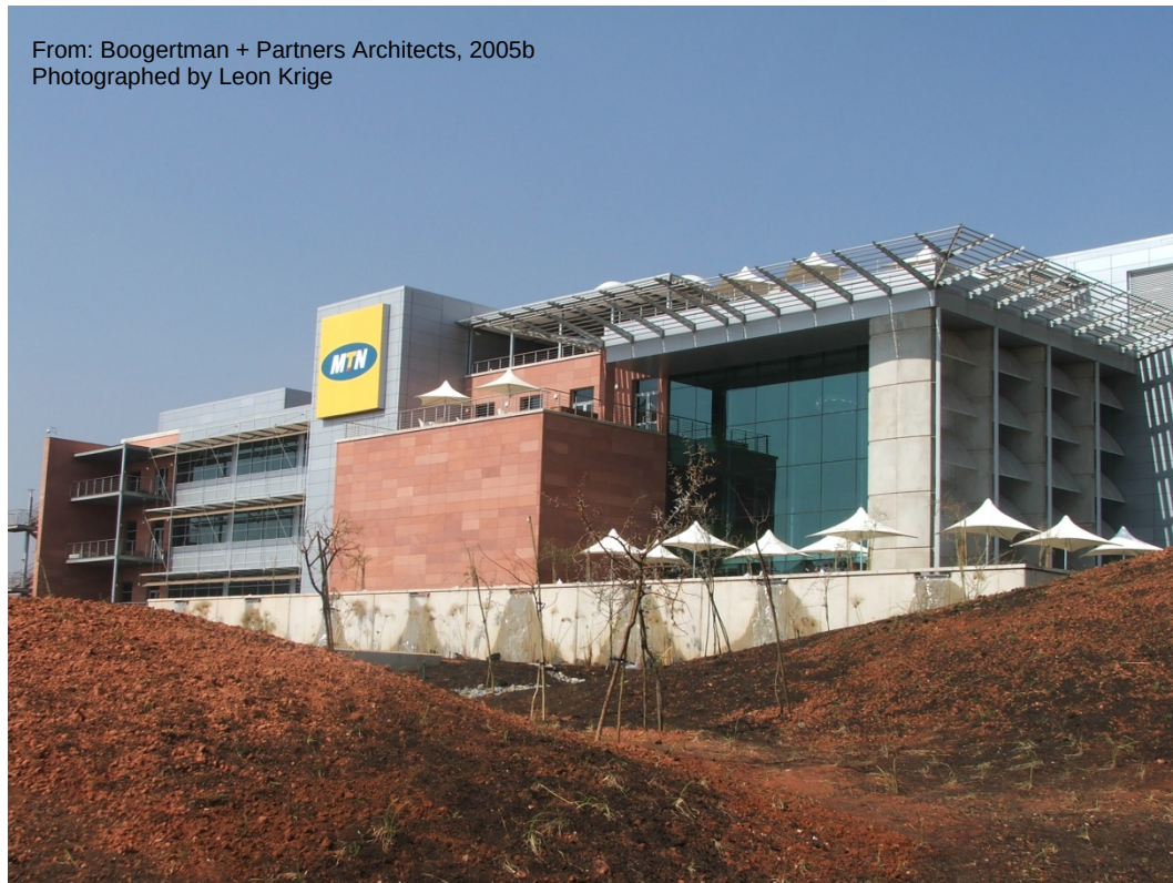
Figure B.2.12 MTN Offices – view of north façade (Boogertman + Partners Architects, 2005b)
