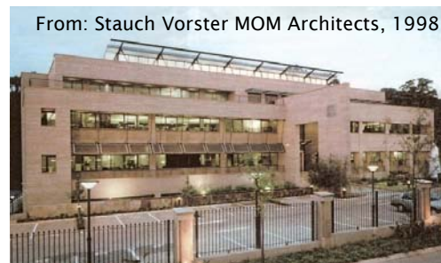
Figure 4.06 South façade of Munich Re-Insurance Centre
