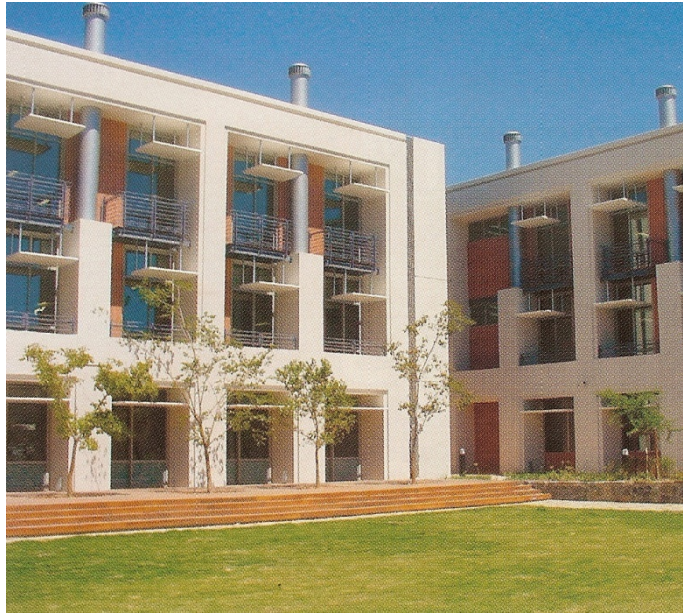
Figure B.4.06 BP Offices – view of north-east façade of building (Noir and Roos, 2005:41)
