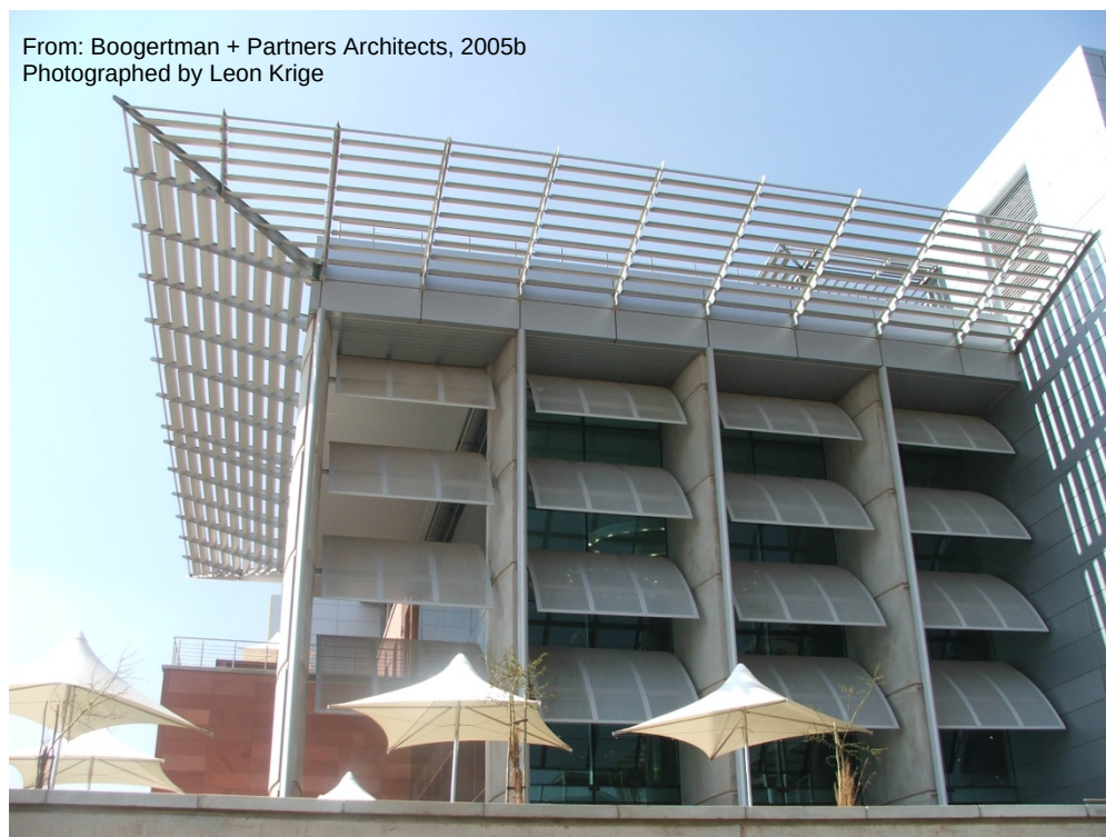
Figure B.2.15 MTN Offices – view of shading devices on west facade (Boogertman + Partners Architects, 2005b)
