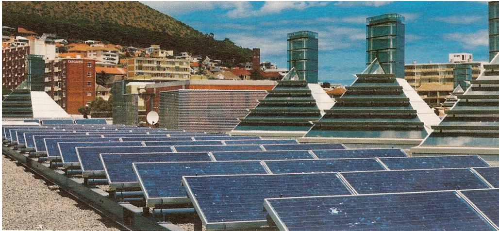
Figure B.4.11 BP Offices – view of roof lanterns and photovoltaic panels on roof (Kruger Roos Architects, 2004:90)
