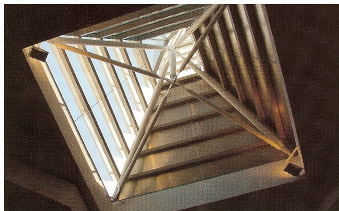
Figure B.4.13 BP Offices – interior view of roof lanterns on roof (Noir and Roos, 2005:39)
