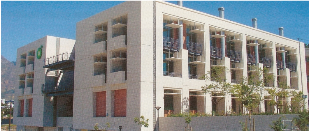
Figure B.4.03 BP Offices – view of north-east façade of building (Noir and Roos, 2005:40)
