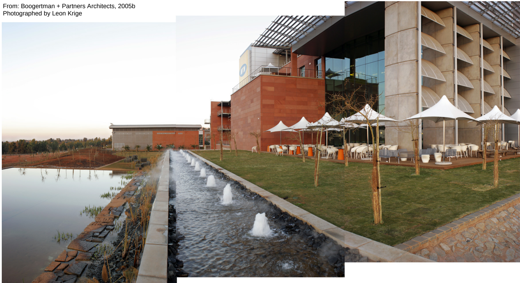
Figure B.2.08 MTN Offices – panoramic view of north and west façades (Boogertman + Partners Architects, 2005b)
