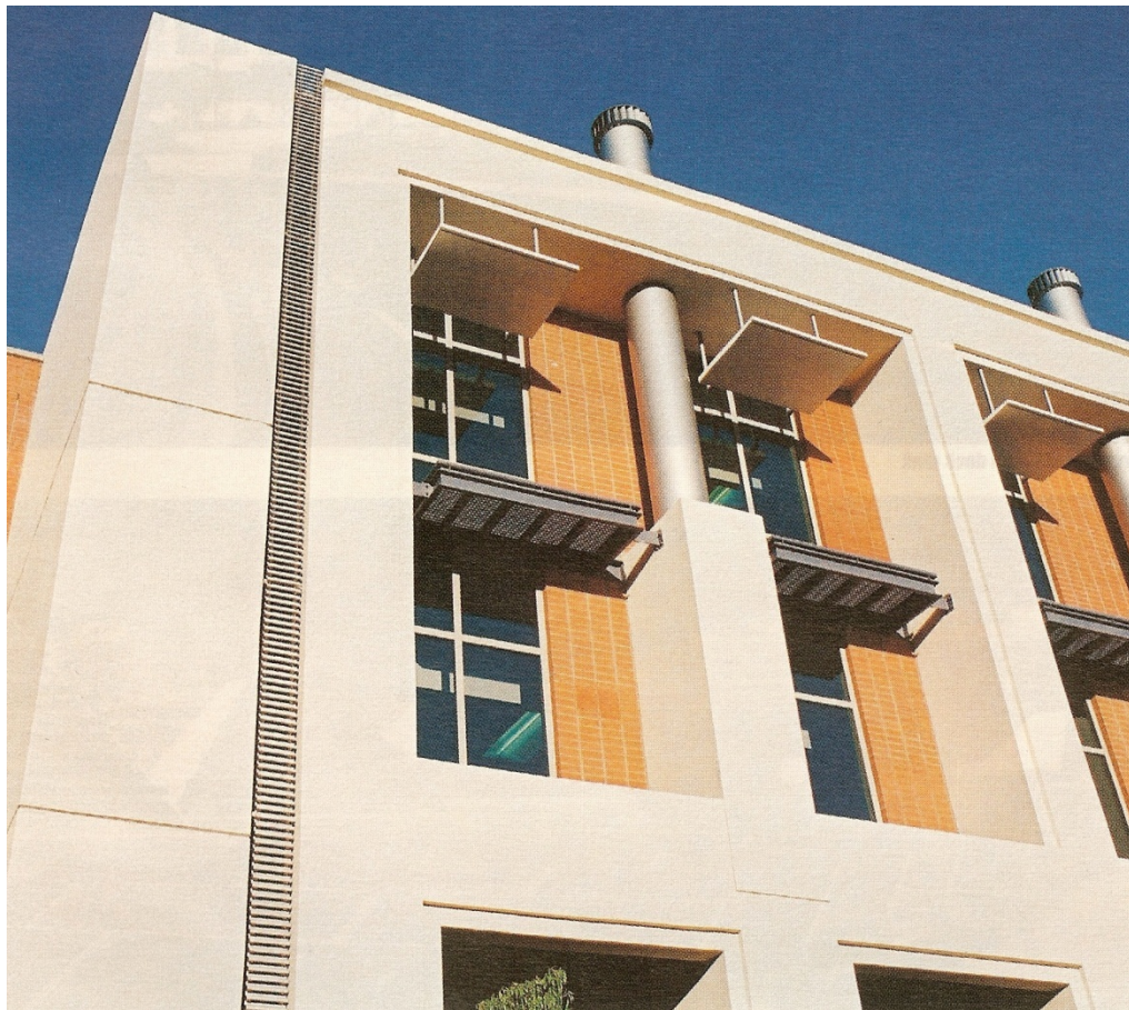
Figure B.4.07 BP Offices – detail view of light shelves, façade shading devices and passive-ventilation turbines (Kruger Roos Architects, 2004:89)
