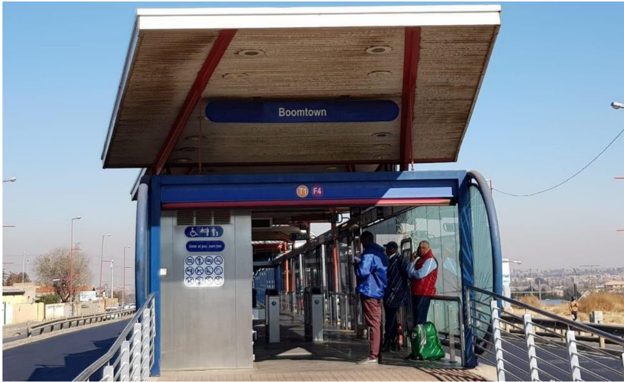
Figure 19: Rea Vaya Station (Photo by Chabalala, 2019)
