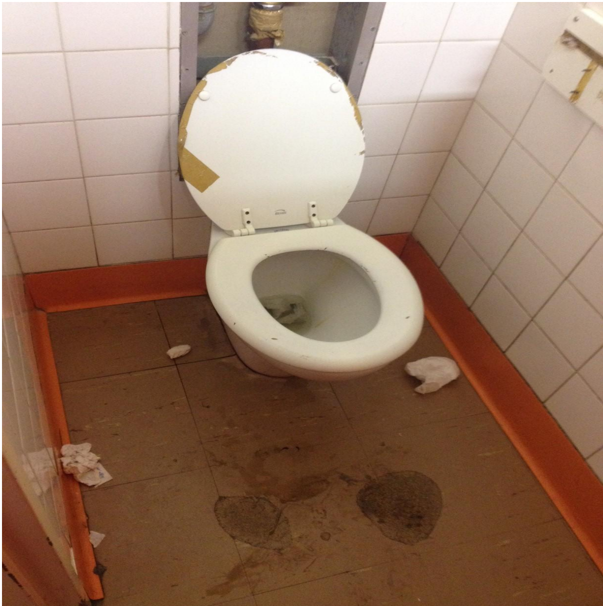
Photograph no. 4: Female toilet
