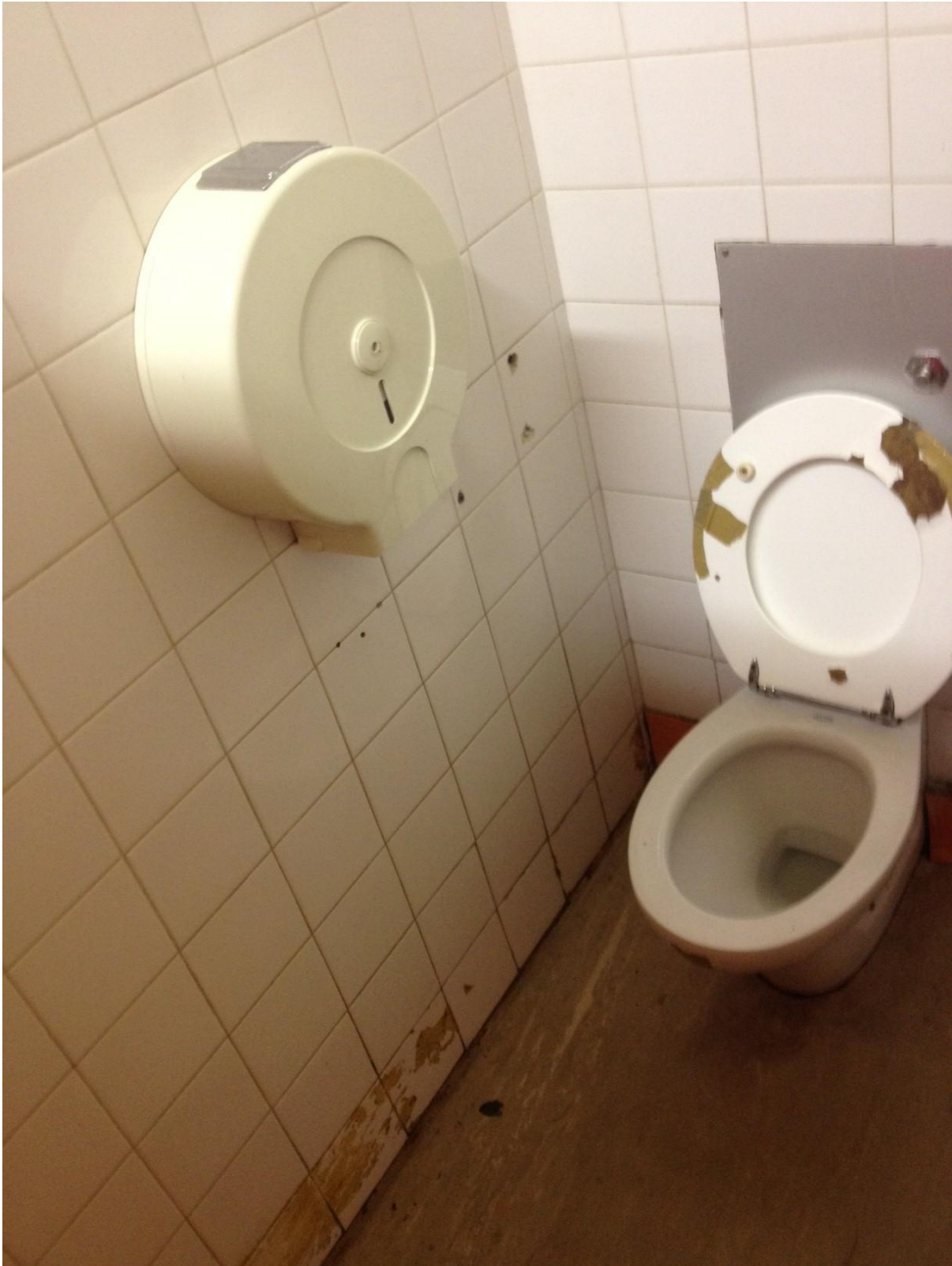
Photograph no. 5: First male toilet
