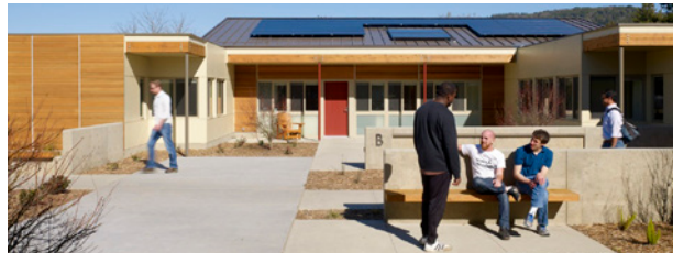
figure 64a: exterior view (ArchDaily, 2013)
