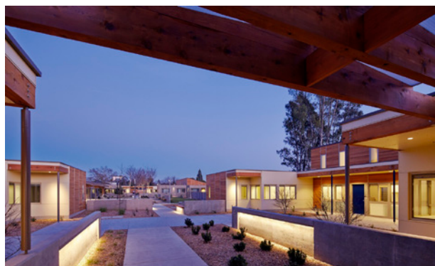
figure 64d: residential building views (ArchDaily, 2013)
