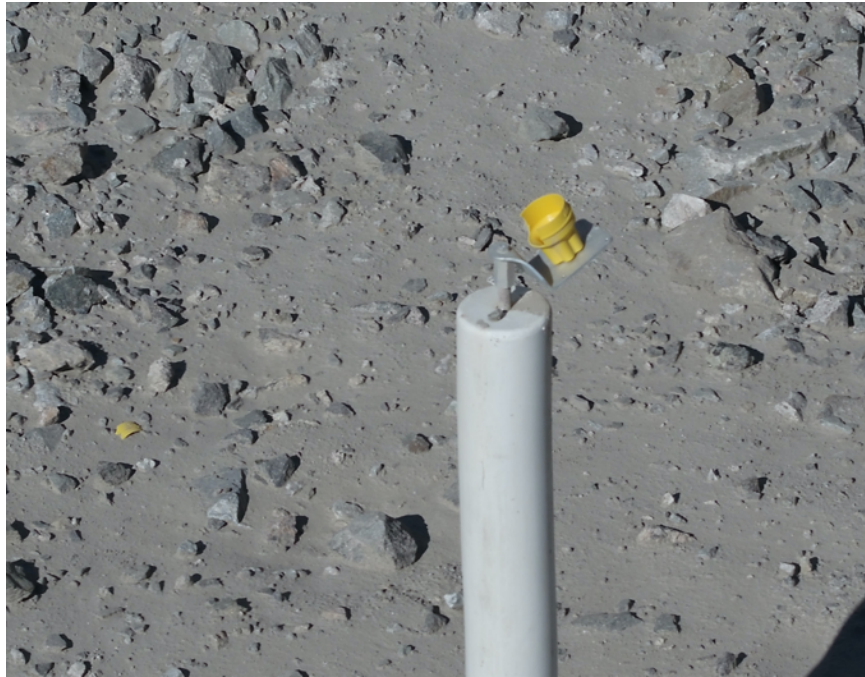
Figure 4-17: A damaged prism and deformed prism structure (RUL Internal Data, 2022).
