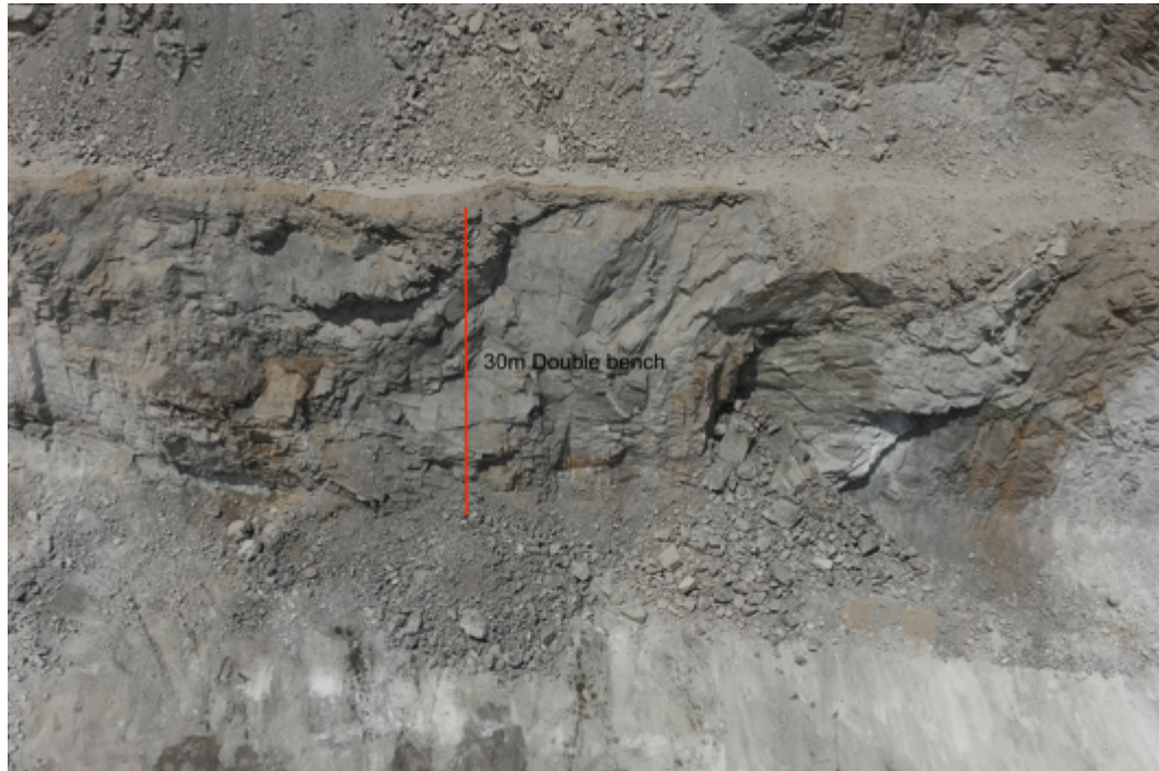
Figure 4-1: An image of a damaged highwall (Aero Vision Drone Services, 2022).
