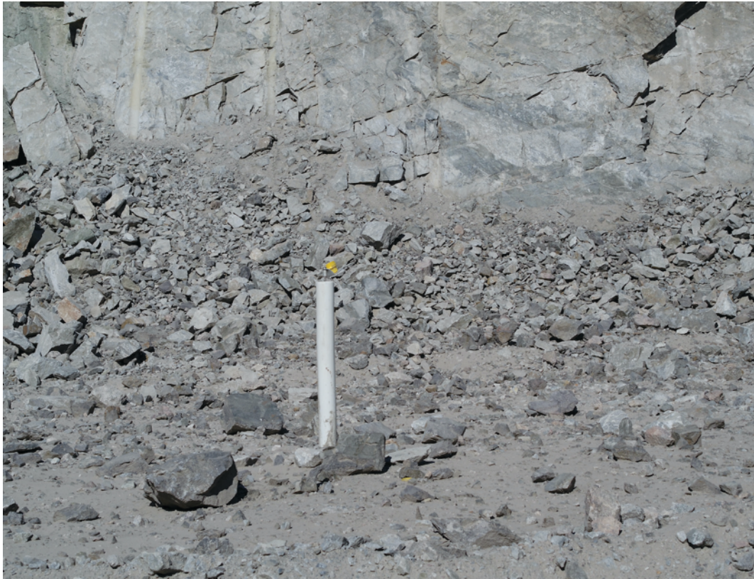
Figure 2-2: A prism installed on a pole grouted into the bench floor (Source: RUL Internal Data, 2022).
