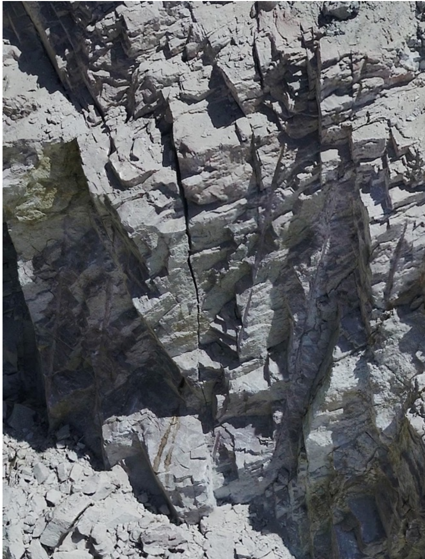
Figure 5-4 A UAV image of a large crack in the highwall (Aero Vision Drone Services, 2022).
