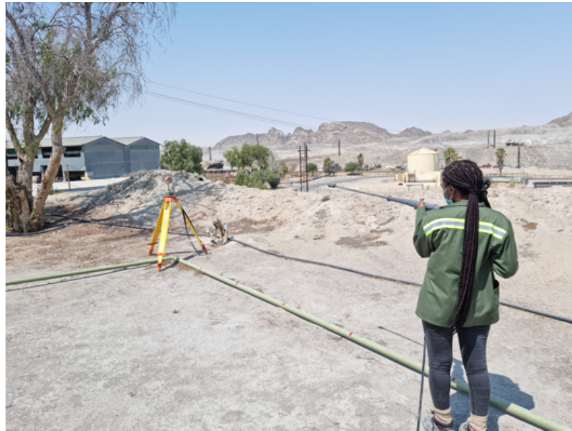
Figure 3-12: The cleaning process, with the nozzle at 4 m from the prism. (Aero Vision Drone Services, 2022).
