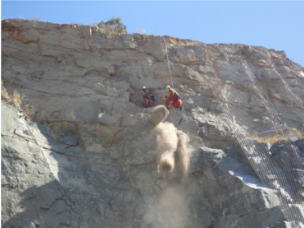
Figure 5-12: An image of abseilers working against a highwall. (Marshal Geotechnical Services, 2018)
