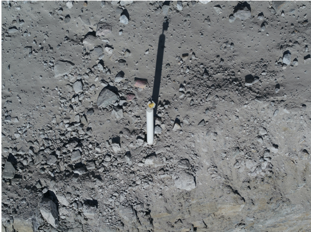
Figure 4-20: A damaged prism near an open edge (highwall) (RUL Internal Data 2022).
