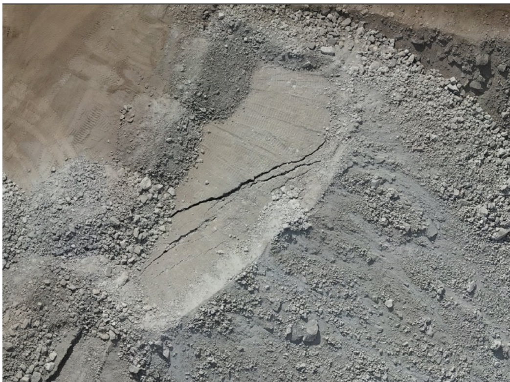
Figure 4-7: Cracks observed on Waste Dump Five (Aero Vision Drone Services, 2022).
