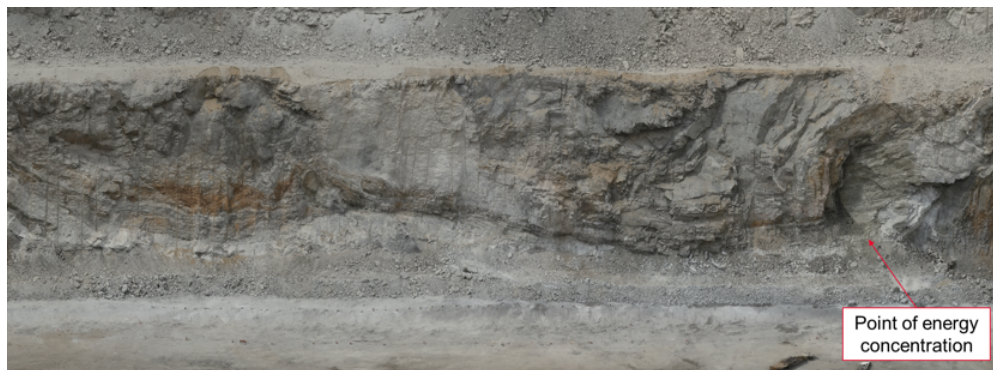
Figure 6-3: An image from a final highwall assessment (Pearce, 2022).
