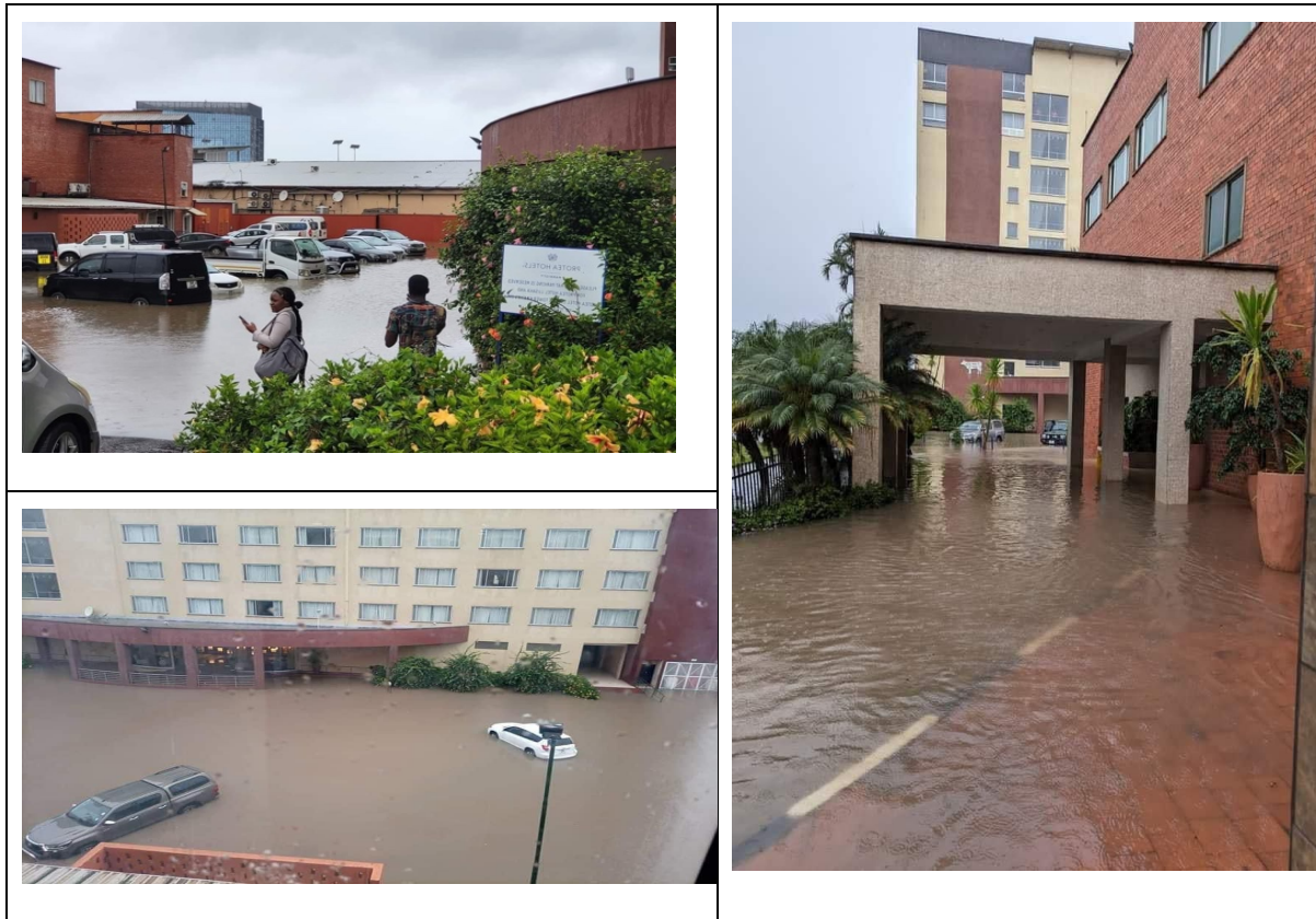
Figure 5.1: Flooded Different Access Points to Protea Hotel Tower at Arcades Shopping Mall.
