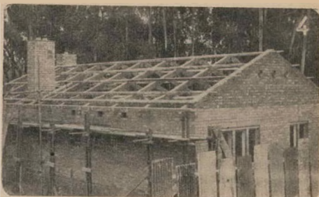
GENERAL VIEW OF HOUSE DURING CONSTRUCTION SHOWING ROOF TRUSSES
