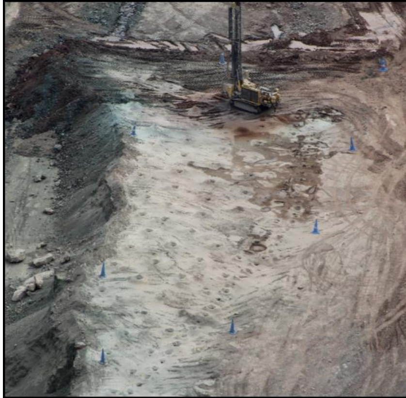
Figure 2.6: Drilling production holes at Orapa mine
