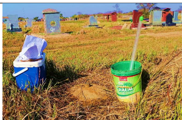
Photo 10: View of MW2 after installation
