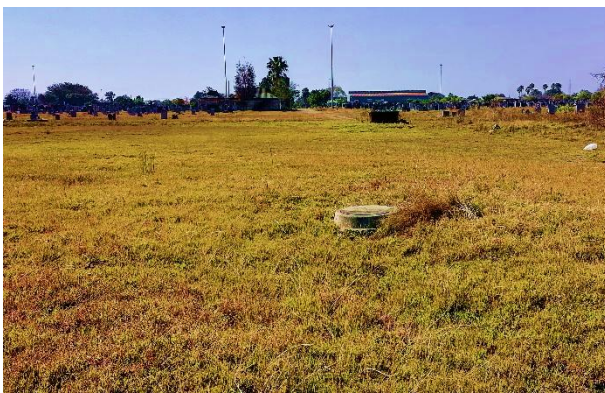
Photo 3: View of sewer utility hole observed on site
