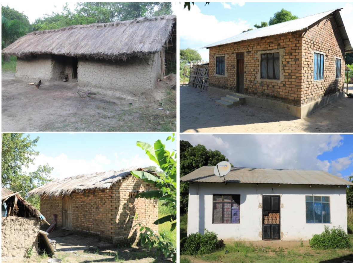
Figure 4.2: Pictorial representation of typical local house types in the study area. Top left - a house with grass thatch roofing with mud walls; top right - a house with corrugated iron roof and brick walls not plastered on the outside, and sometime also not plastered on the inside, bottom left - a grass thatch roof with brick walls not plastered on the outside, and sometime also not plastered on the inside, and bottom right - a house with iron sheet roofing and plastered brick walls. A variety of window and door designs are evident.
