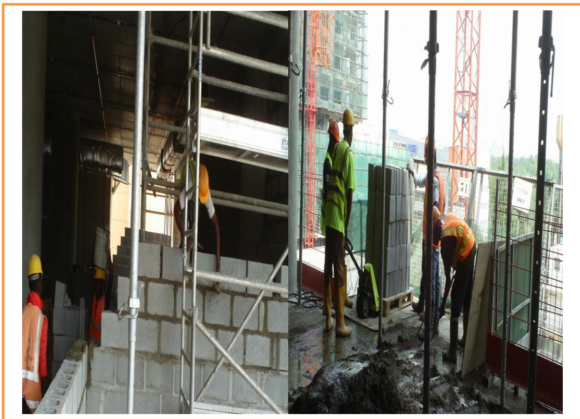
Figure 4.4: Mortar mixing (1:4) with 10 mm mortar joint on Blockwork
