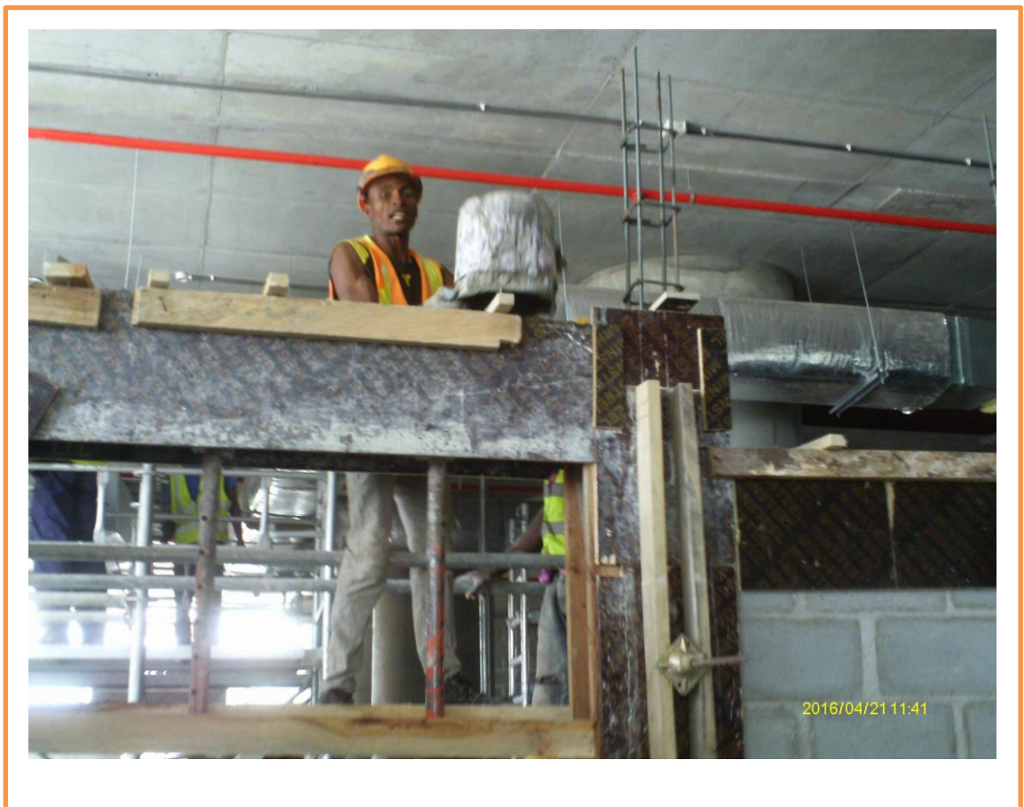
Figure 4.6: U-block casting with good vibration of the Concrete
