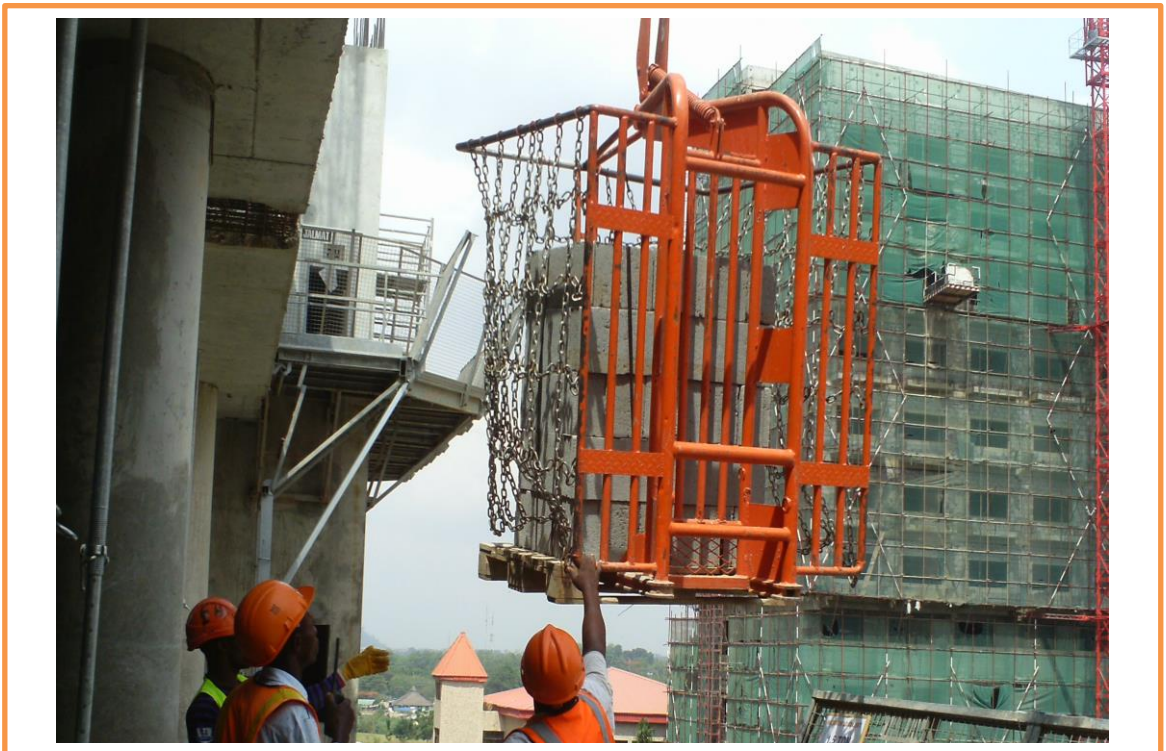
Figure 4.7: Transportation of Blocks via Crane to Height of Work
