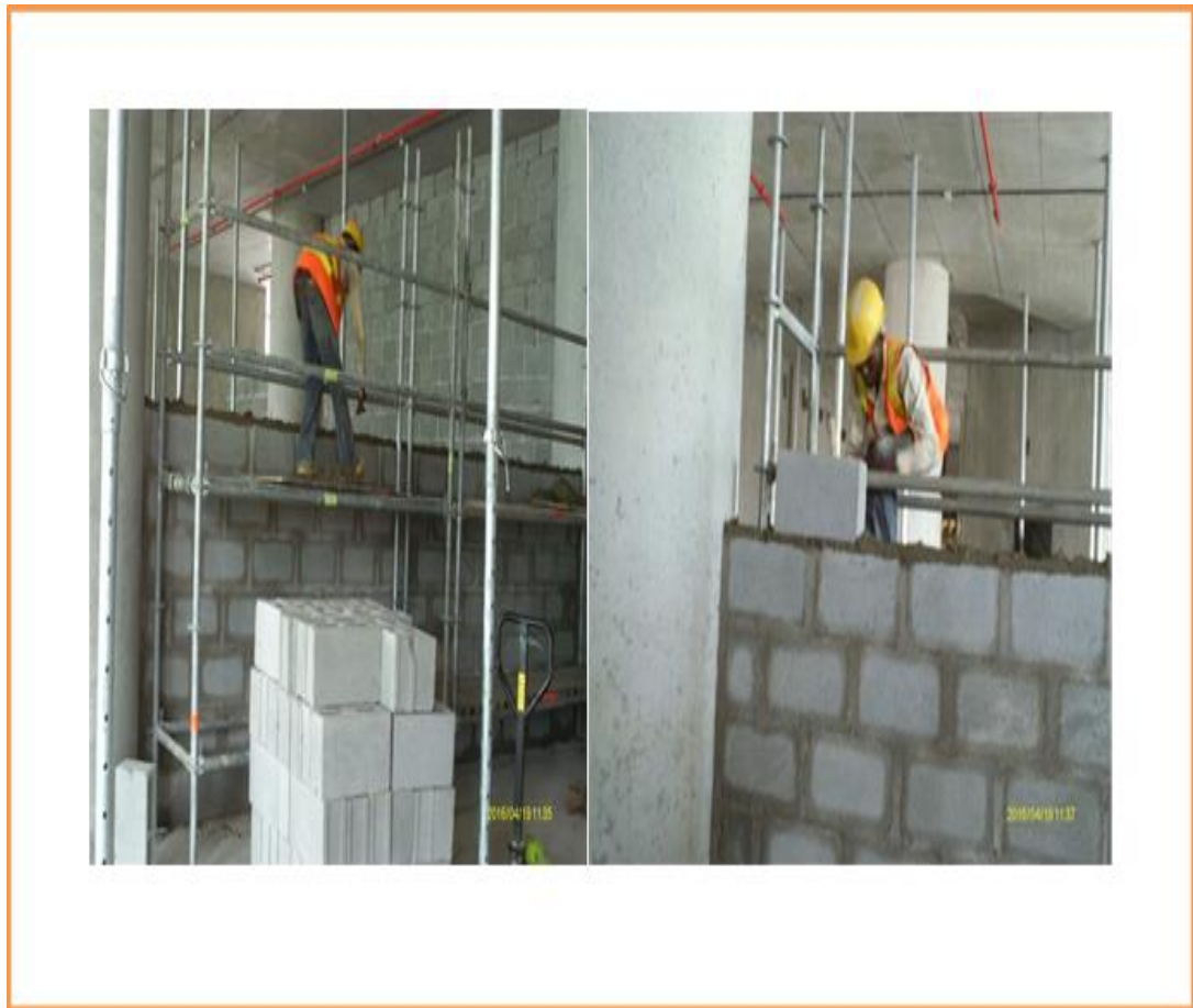
Figure 4.5: Typical Block Wall Erection with Wall Stiffener
