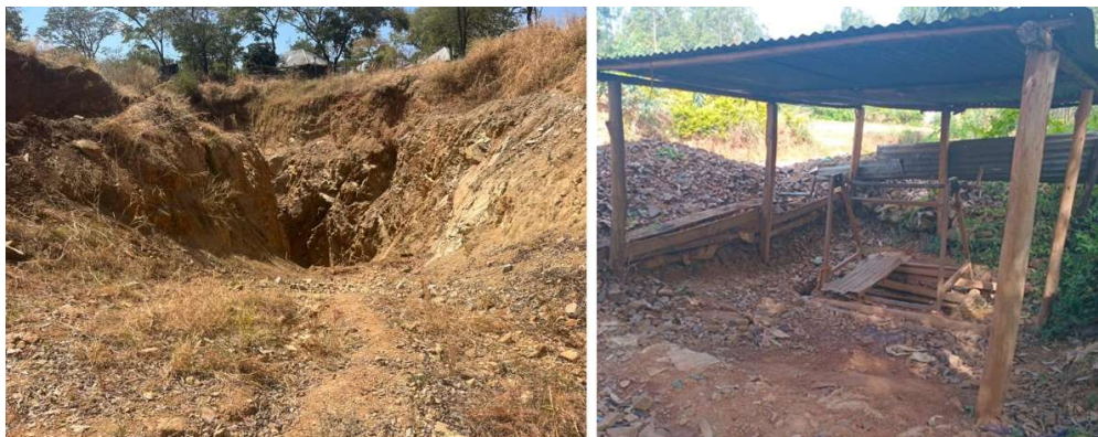
Figure 17: Open and unfenced shafts
