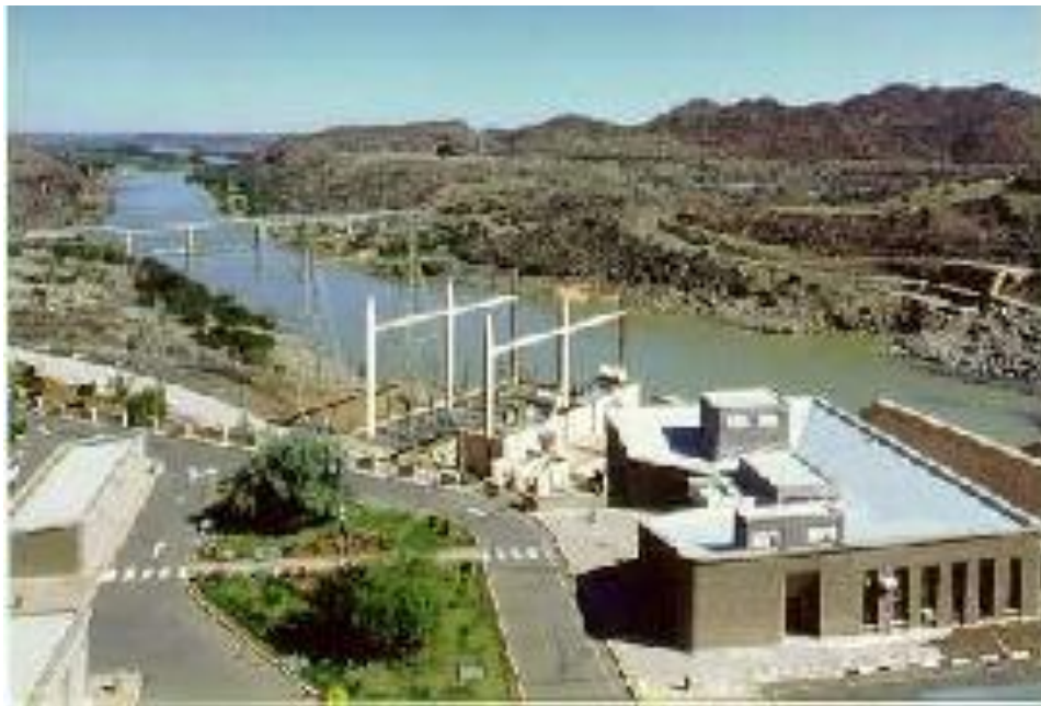
Figure 40 - Vanderkloof Hydro Electric Power Station
