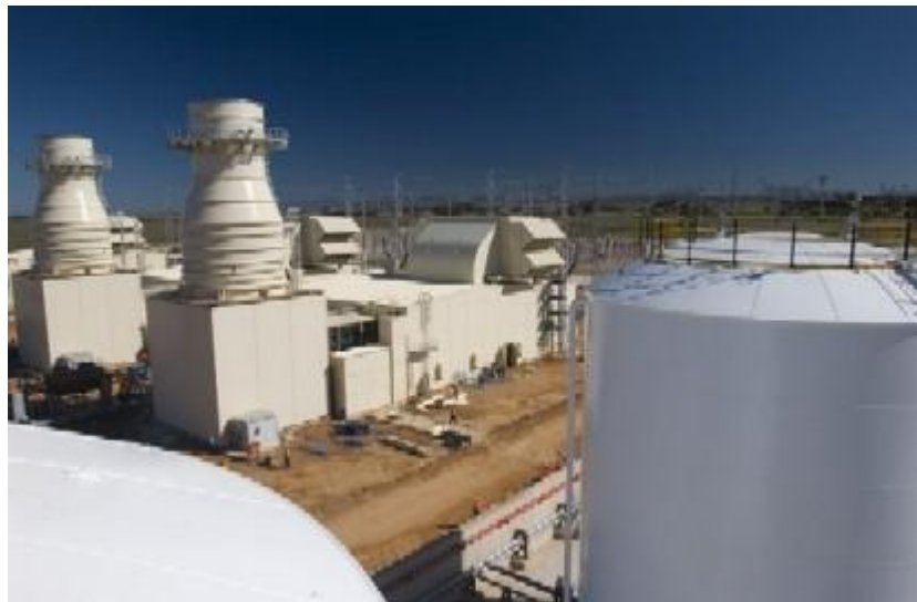
Figure 34 - Gourikwa Open Cycle Gas Turbine Plant
