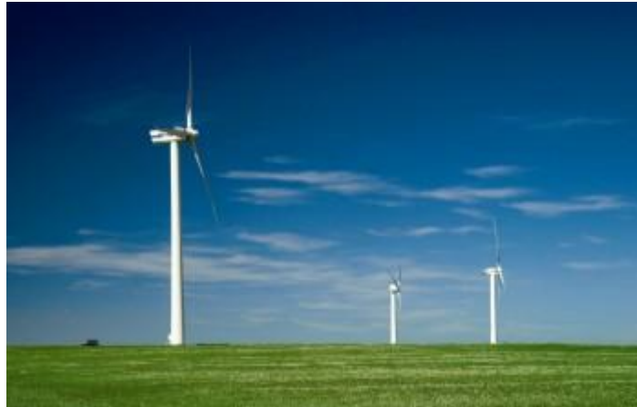
Figure 41 - Klipheuwel Wind Energy Facility
