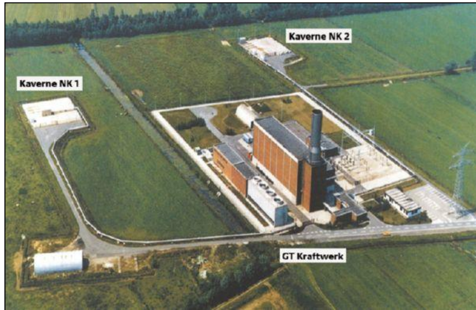
Figure 18 - Aerial View of the Huntorf Plant (BBC, 1990)
