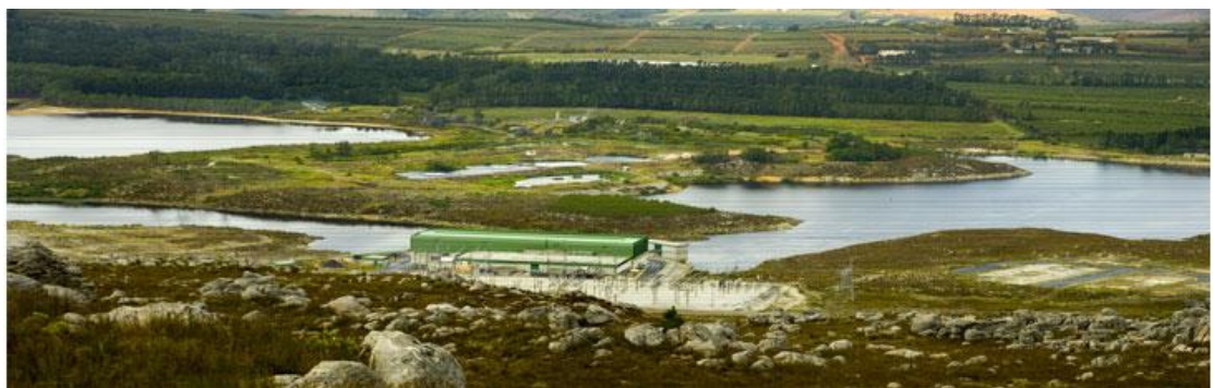
Figure 36 - Palmiet Pumped Storage
