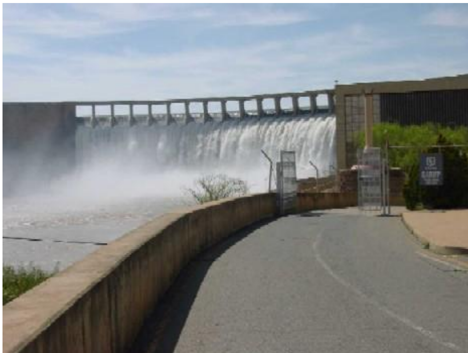
Figure 39 - Gariep Hydro Electric Power Station
