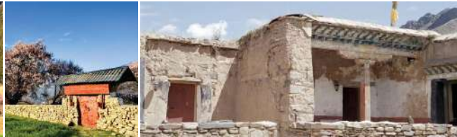
Fig 1.12 Below Edited Photograph Local Stone Walls, Sasong Village (Author, 2023)
