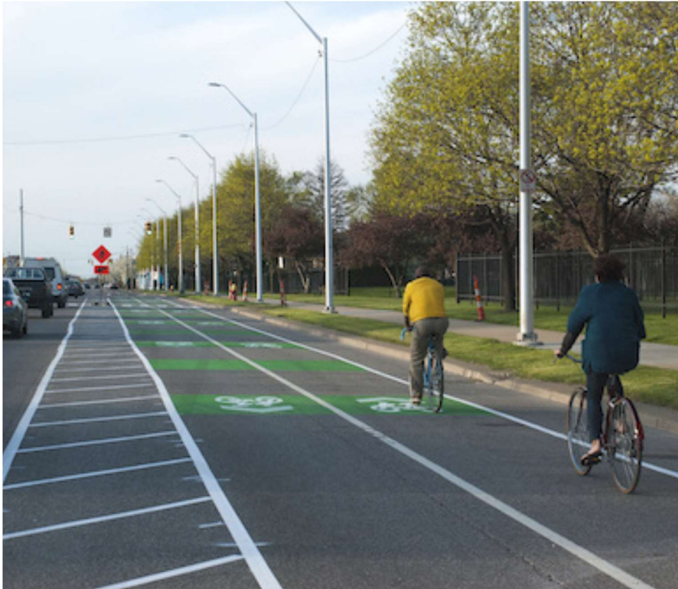
FIGURE 35: BIKEWAY DEMONSTRATION - TEMPORARY LANE REALLOCATION (TU GUIDE, 2016)
