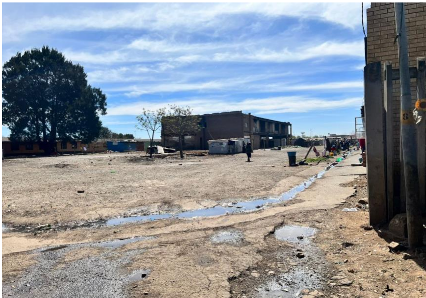
Image 2: Broken down sewage system at Mshayazafe Hostel, Thokoza
