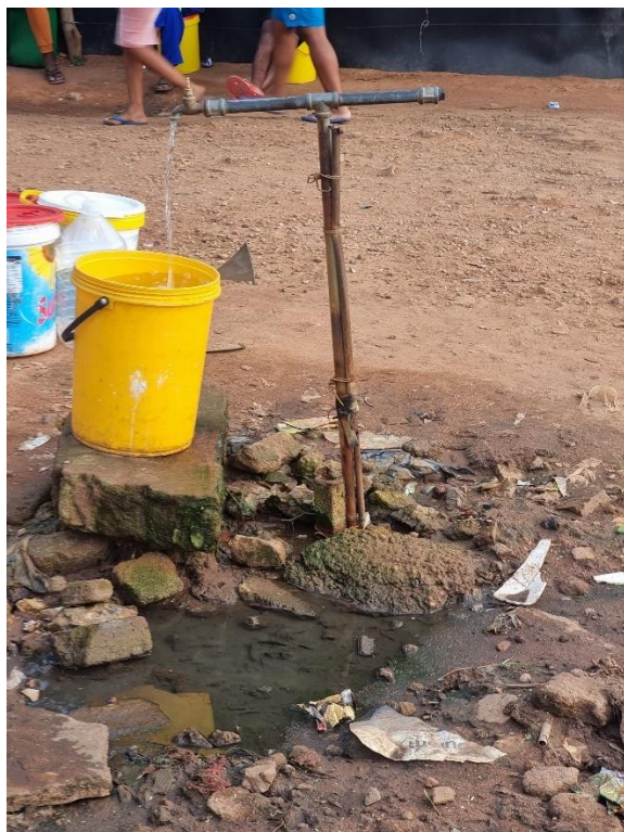
Figure 9: Communal standpipe for water supply in the Mahlakong informal settlement
