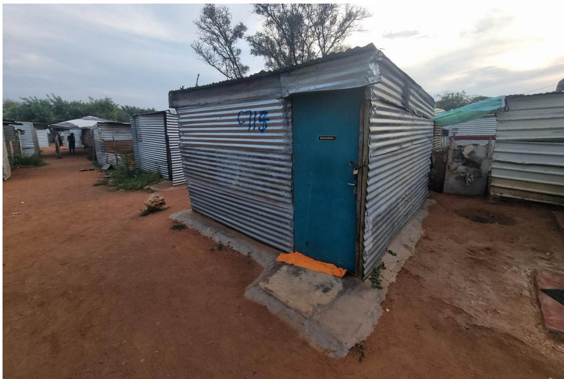
Figure 13: A dwelling in the Mahlakong Settlement with a stand number inscribed using blue spray paint.
