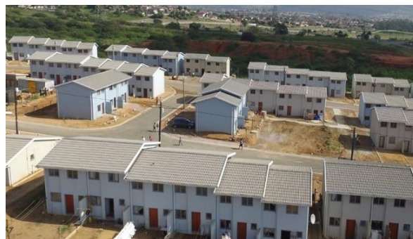
Figure 7: Cornubia human settlements project with double storey IRDP housing units (SABC, 2019).
