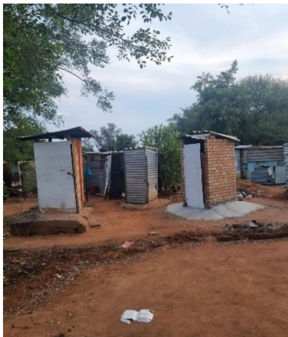
Figure 11: Multiple self-constructed pit latrine toilets clustered together in a section of the Mahlakong Informal Settlement belonging to various households.
