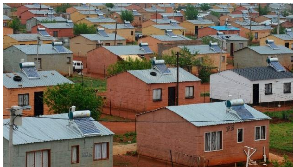
Figure 6: The commonly seen design of IRDP housing settlements in South Africa (polity, 2017).
