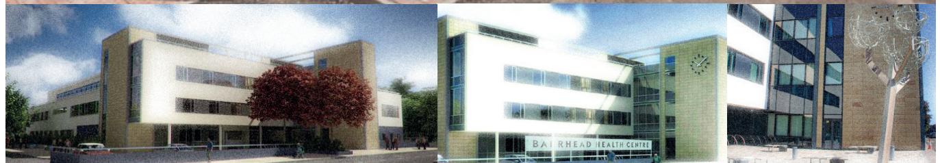
Fig. 82. Exterior view and building aesthetic (www.vimeo.com; www.gleniffermedical.co.uk; www.drookitagain.co.uk)
