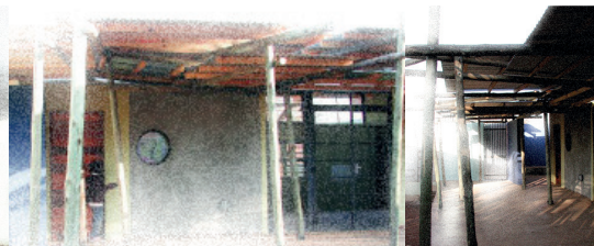
Fig. 63. Randomly ordered pergola timber posts ( www.wolffarchitects.co.za )
