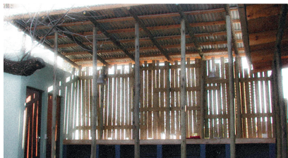
Fig. 61. North verandah & urban corridor ( www.wolffarchitects.co.za )
