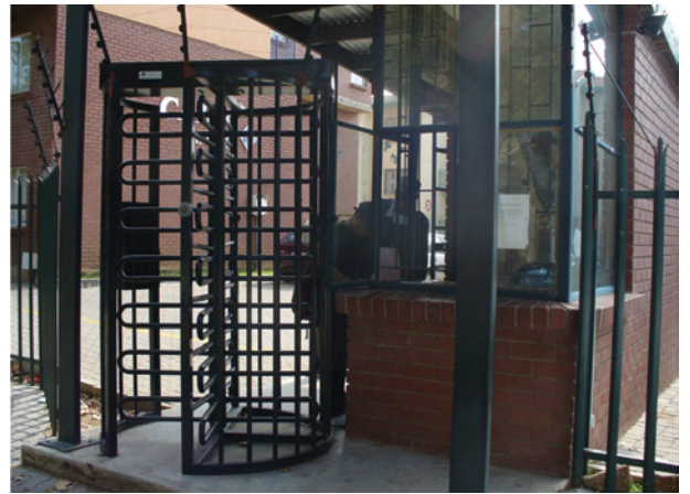
FIGURE 29: Entry into this affordable housing project is controlled and pedestrians have to pass through security and either have a resident's card or state the purpose of their visit.
