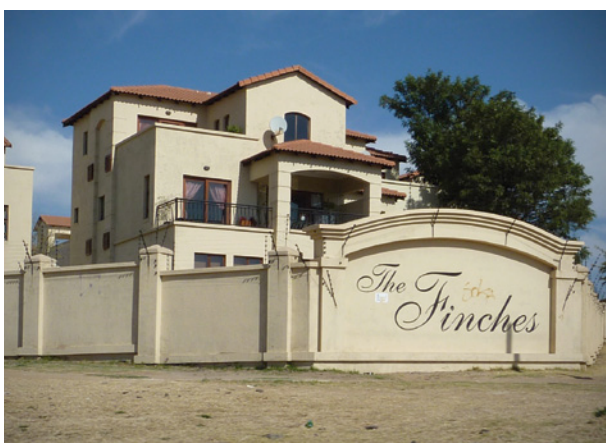
FIGURE 19: A secure gated townhouse located in the far northern suburbs of Johannesburg. Access is controlled and the entire perimeter is protected by a wall and electric fencing. The architectural style of the wall also contributes to the identity of the complex.
