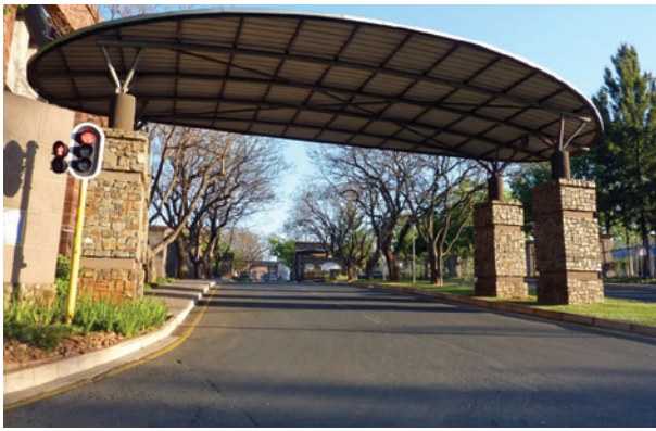
FIGURE 32: Entrance to secure office park near Wanderers, Colette Drive
