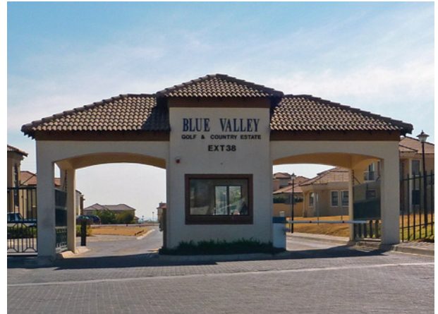
FIGURE 13: Side entrance to a large luxury estate in the north of Johannesburg. This estate has more than one entrance controlled by private security guards and boomed gates.
