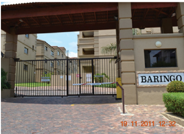
FIGURE 26: This image indicates a three storey walk-up, covered by a blank frontage. The security measures are quite stringent with security gates, a boom and a security code upon entrance. This gated townhouse is situated within the northern suburbs of Johannesburg.
