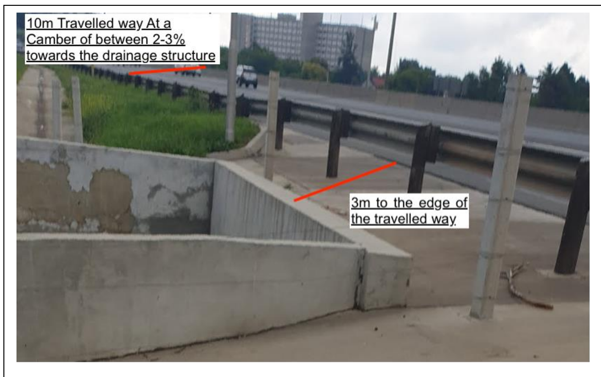
Figure 5.9: Inlet of the Drainage Structure at the Study Area.
