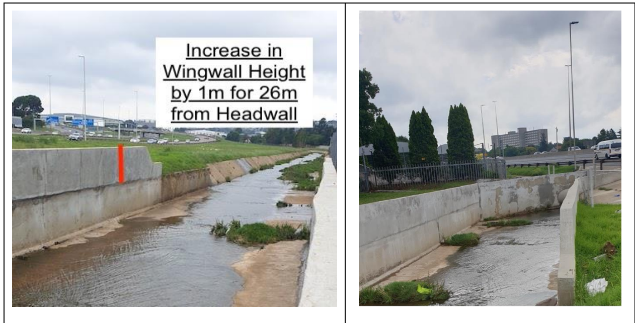
Figure 3.5: Upstream of the channel also showing the extent of the increased wingwalls (see A and B in Figure 3.4).
