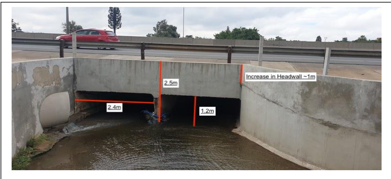
Figure 3.2: Showing the inlet at the drainage structure with a clear construction line on the wingwall indicating when increased height (See B in Figure 3.4)
