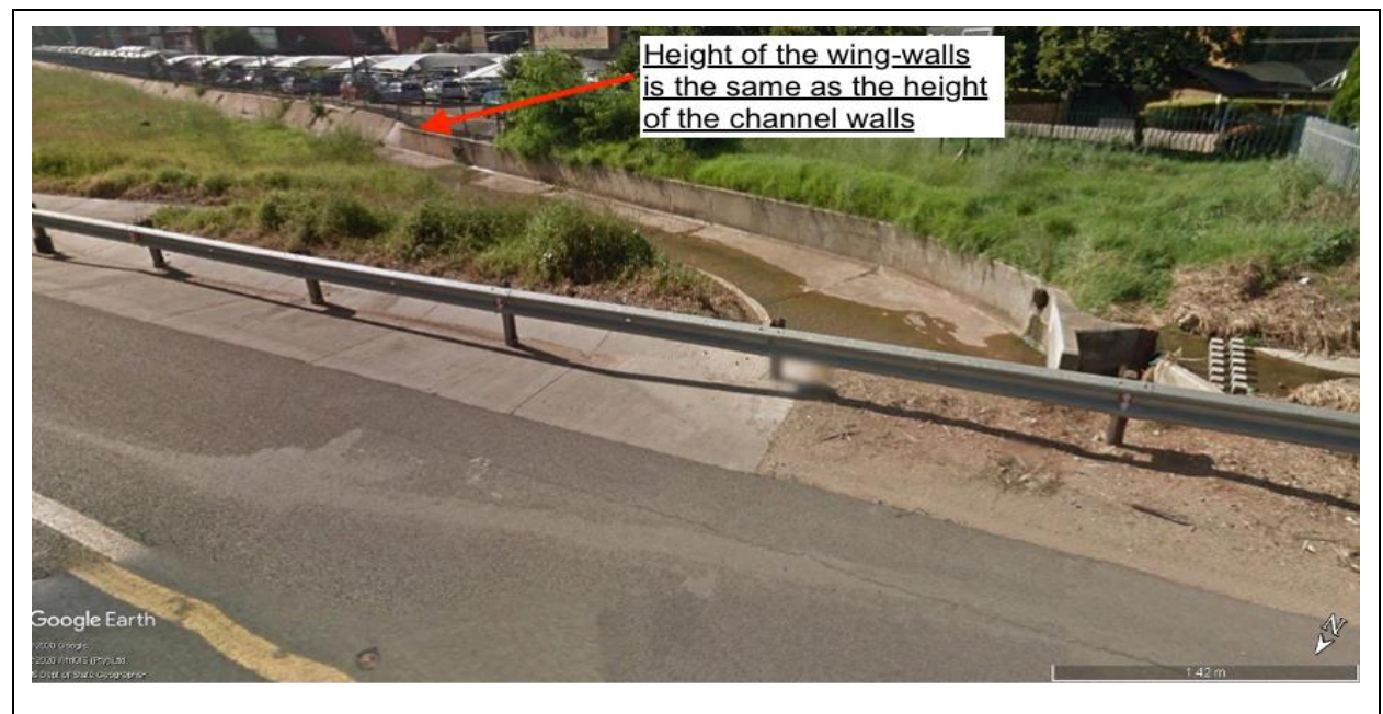
Figure 3.6: Upstream of the Drainage Structure Before Upgrades (Google Earth 2018)
