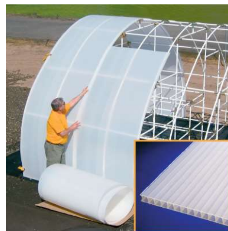
III. 7 Installer placing Polycarbonate sheet over green house. https://secure.img1-fg.wfcdn.com/im/16358486/resize-h600-w600%5Ecom-pr-r85/5440/5440811/PRO+5mm+Polyethylene+Panel.jpg
