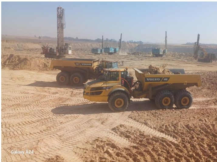
Figure 4.12: ADT hauling to the dumping area
