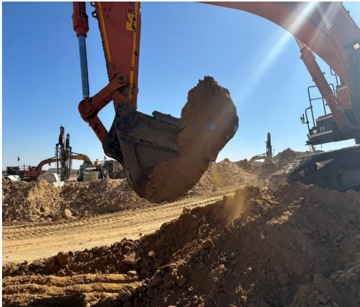
Figure 4.11 : Excavator loading subsoil
