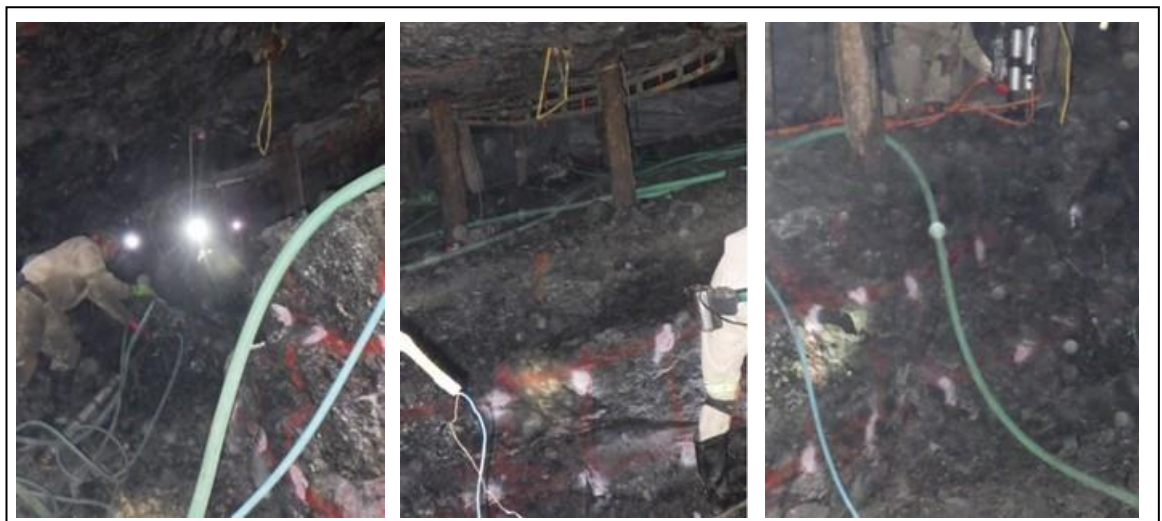
Figure 5-31: Alternative trench and retreat method being implemented.
