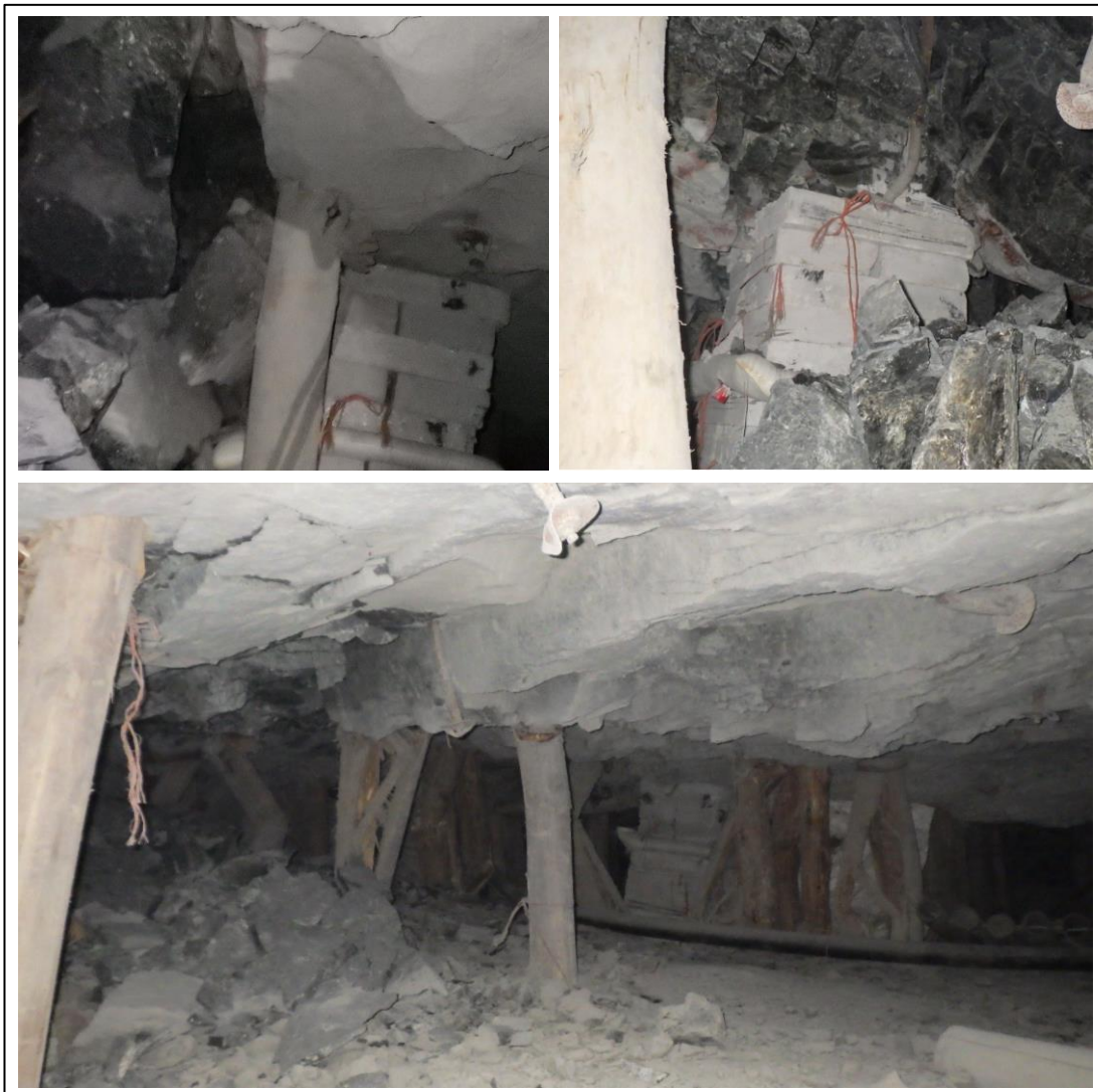
Figure 5-13: Photographs of Dura-Paks arresting the propagation of large-scale collapses (Impala Platinum, 2017)
