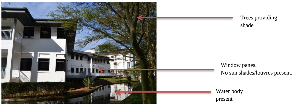
Figure 20: Building components on the northern façade that influence the micro climate.
