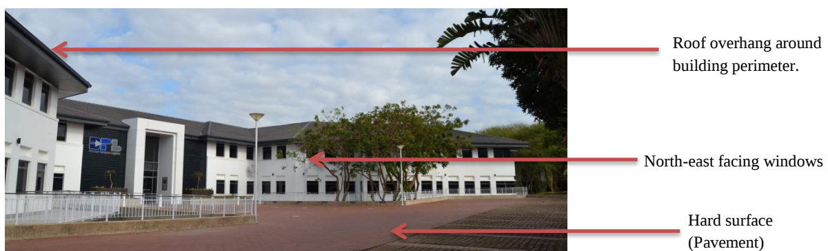
Figure 19: Building components on the eastern façade that influence the micro climate.
