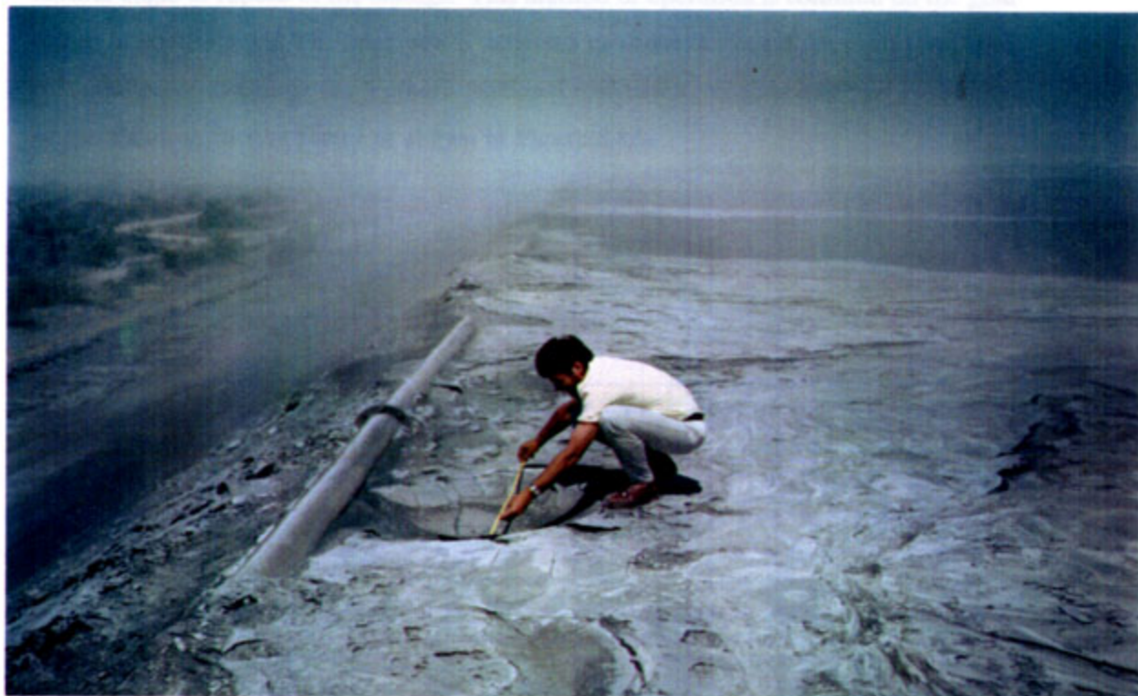
FIGURE 8.43 : PHOTOGRAPH OF THE SPRAY-BAR DISCHARGE PIPE AT PERING MINE
