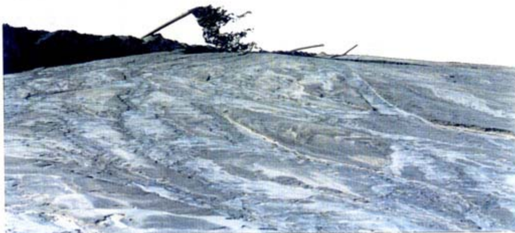
FIGURE 7.28 : PHOTOGRAPH OF A TYPICAL DISCHARGE ON THE MAGNETITE DAM
