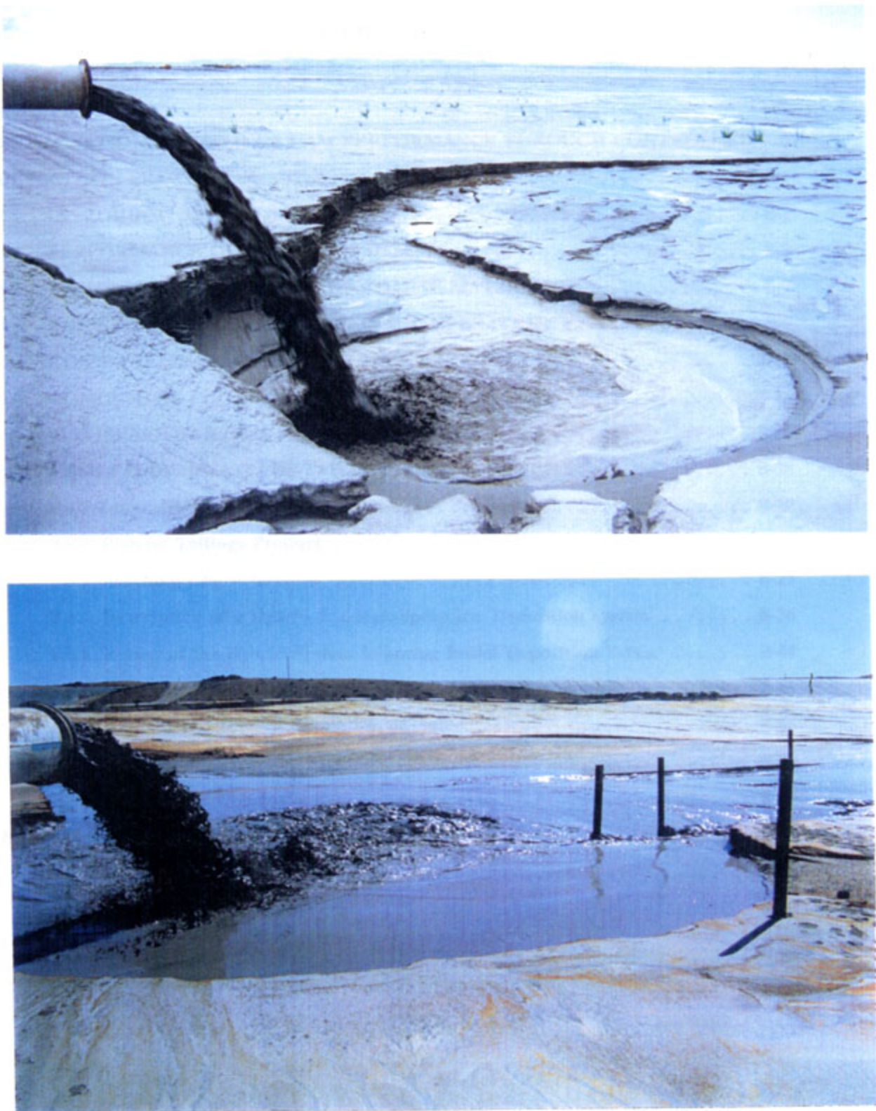
FIGURE 7.34 : PHOTOGRAPHS SHOWING TYPICAL DISCHARGE STREAMS AND THEIR EFFECT ON THE PLUNGE POOL VELOCITY
