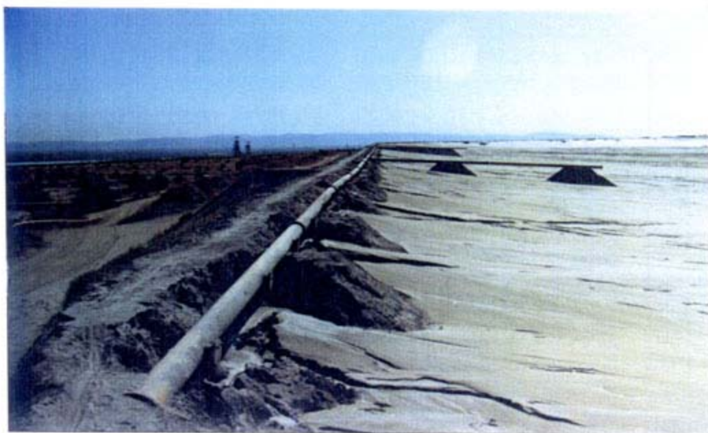
FIGURE 8.32 : PHOTOGRAPH ILLUSTRATING TYPICAL SPECTACLE PLATE FAN SPRAY OPERATION
