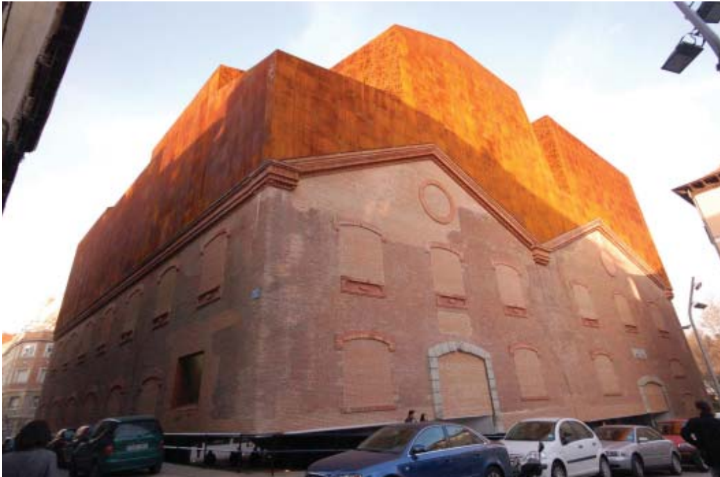
8-1. to double the museum's volume, a rustic steel cladding to blend with the old building's old brick. The new structure sits on the existing building though supported by the well hidden steel structural system. (Etherington 2008)
