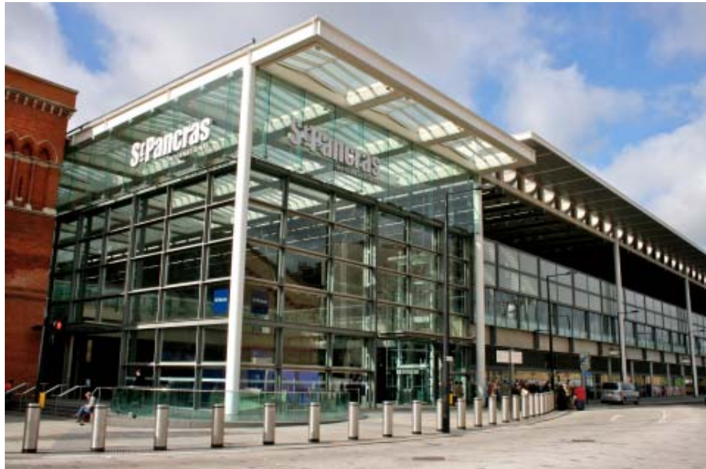
5-25. entrance view of glass and steel (van Uffelen, C, 2010)
