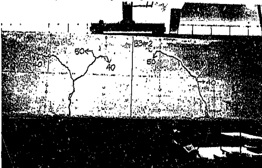
Figure 6.5 Crack pattern of the fully prestressed beam from series B (post tensioned unbonded strands)
