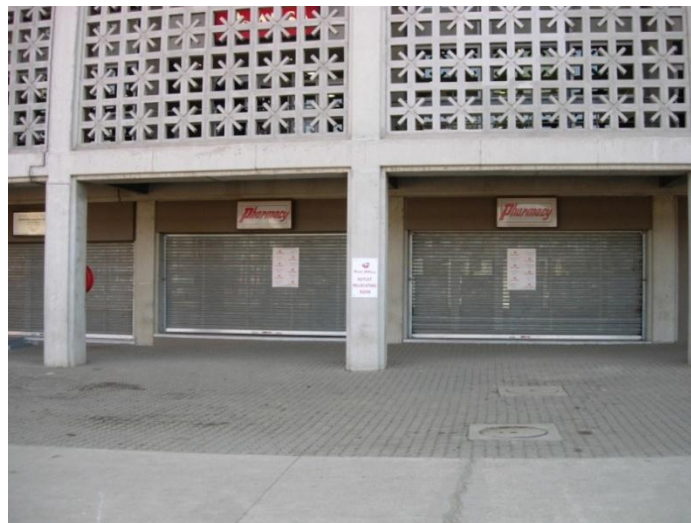
Figure 41 (2008): Concrete crosses symbolising democracy adorn the walls above empty, shuttered shops. Photo: Naomi Roux.
