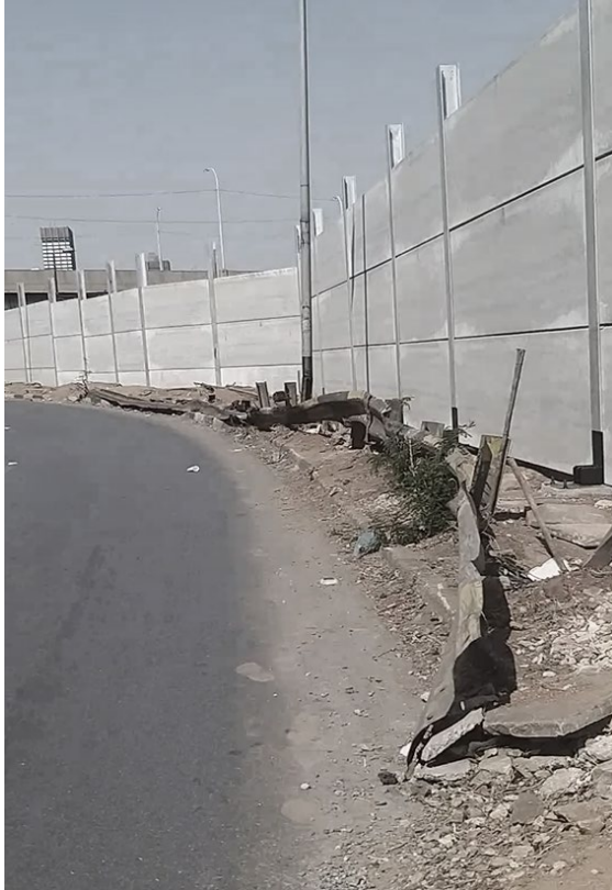
Figure 44: Most concerning addition to the site is the 4m wall on the edge of the tracks which further isolates the site from its surrounds (Author, 2023)
