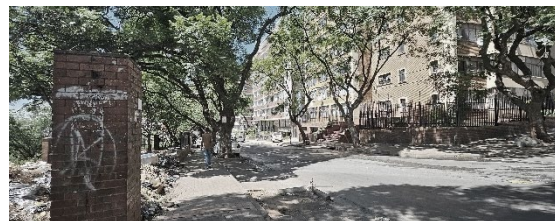
Figure 59: Deterioration and litter, Berea Point Park (Author, 2024)
