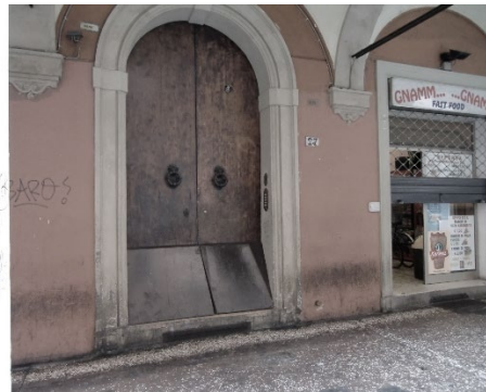
Figure 55: New protective mechanism at door of an old entrance way, 2009 (photograph by Arnaud Elfort and Guillaume Schaller of Survival Group. Project “Anti-sites”)
