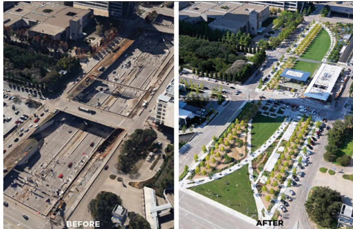
Figure 119: Reclamation of the space above 8-lane highway, Burnett, J (2013).
