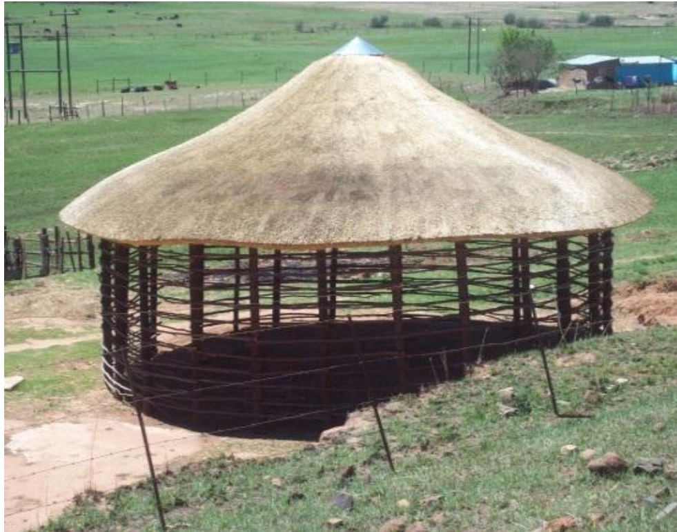
Figure 6.2: A hut under construction: walls yet to be built
