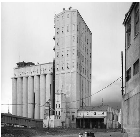
Picture 7.4: The old and new silo buildings
