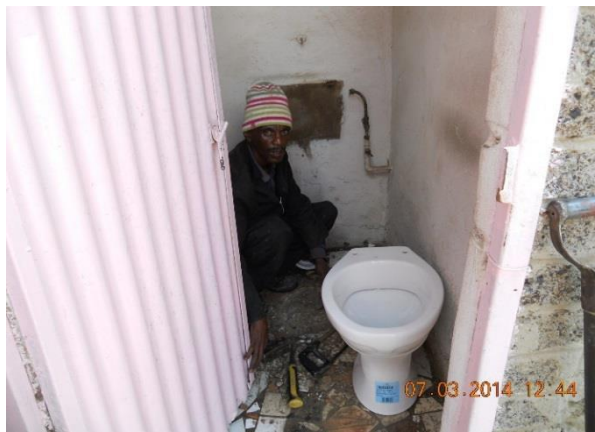
Figure 4.1: Retrofitting of an outside toilet on adjacent properties (pictures taken from: EMM, 2015).
