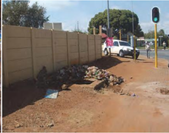
Figure 4.4: Cleaning rubbish from chamber
