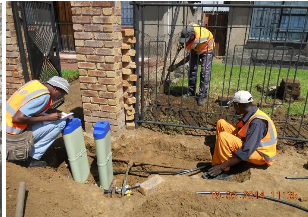
Figure 4.2: The labour team in the process of installing two meters
