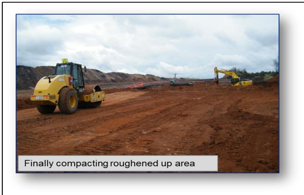
Figure 4-7: The compaction of the backfilled void by the roller in high risk areas.
