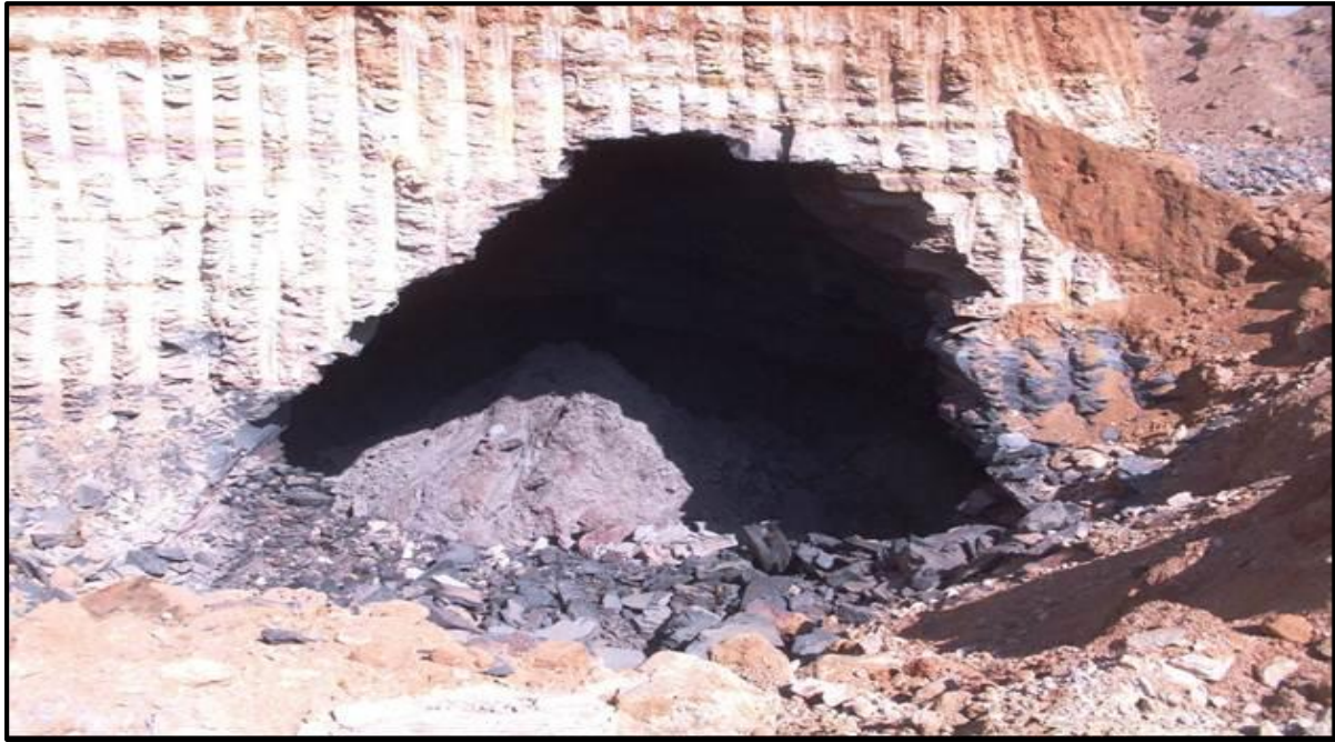
Figure 2-4: Progressive failure of the roof and sinkhole migration to surface.
