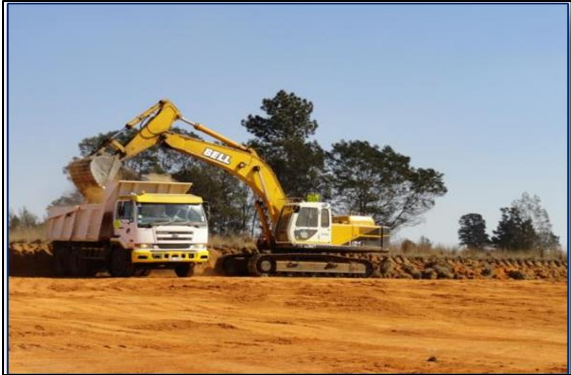
Figure 4-3: Top soil reclamation in areas to be roughened up (High risk).
