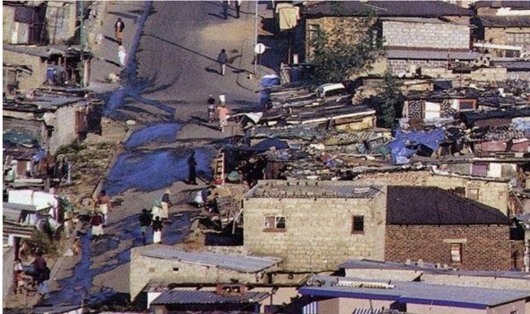
Figure 3.2: Image of deteriorating Infrastructure in Orange Farm
